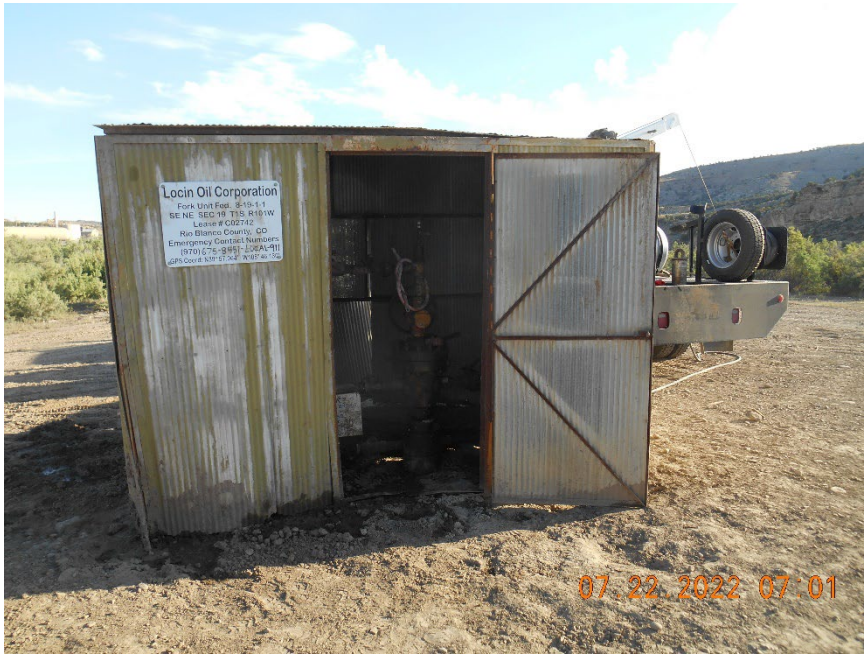
Injection wellhead inside housing during MIT
