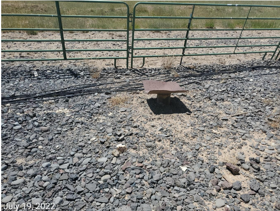
Photo 4: Well marker for the Coury 18-2 well. Marker does not comport with monument requirements, however, marker is located within a string of active wells, does not appear to be interfering with production activities, has been fenced off and not an apparent safety issue.
