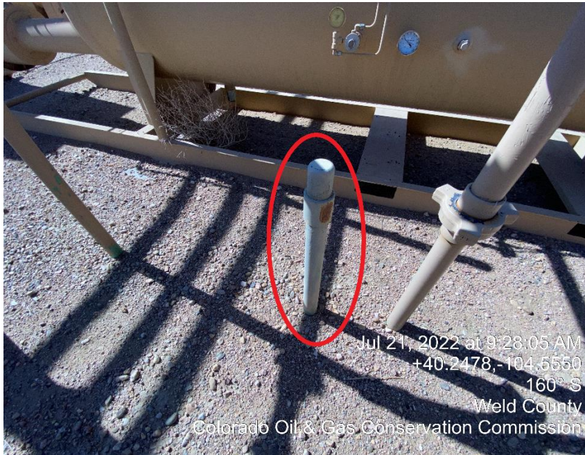
Photo #5 Unmarked Riser
