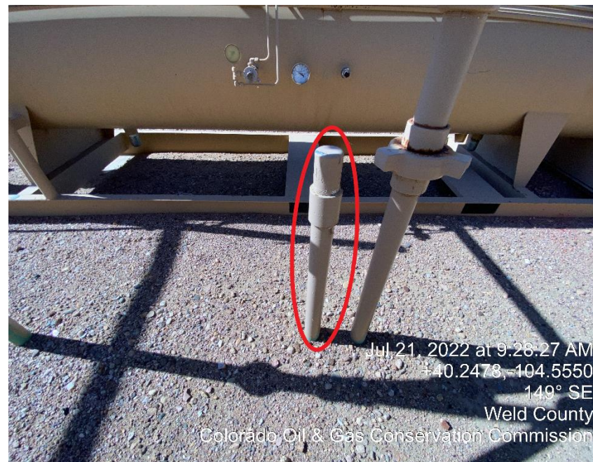
Photo #4 Unmarked Riser
