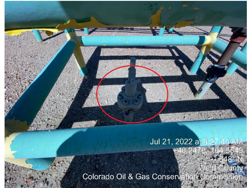
Photo #2 Unmarked Riser
