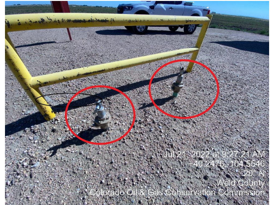
Photo #8 Unmarked Riser
