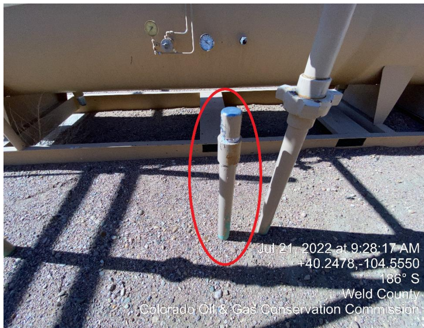
Photo #3 Unmarked Riser
