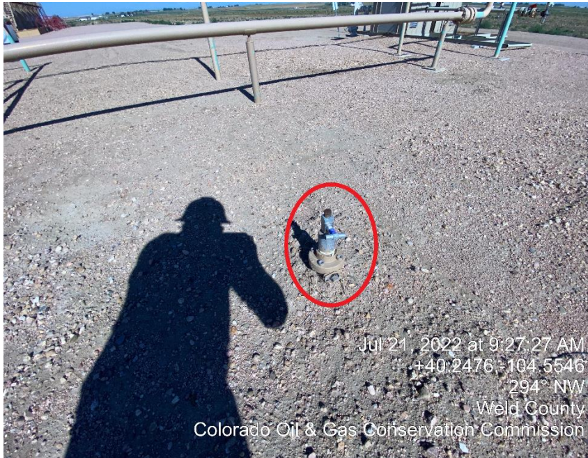
Photo #7 Unmarked Riser
