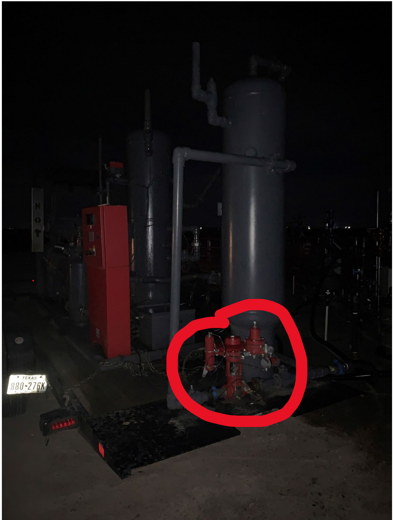
Figure 1 This is what we think failed open and pressured up the pop-off's
