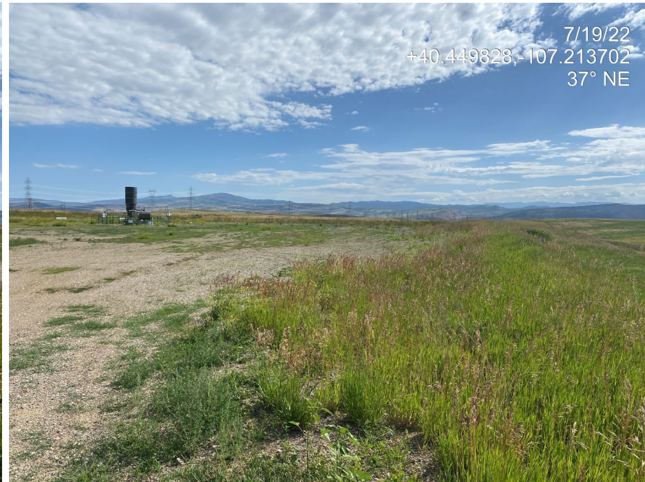
Photo 2. Photo taken from the Location entrance shows an overview of the eastern portion of the Location. Photo shows a portion of the pad not necessary for production operations where interim reclamation is required.
