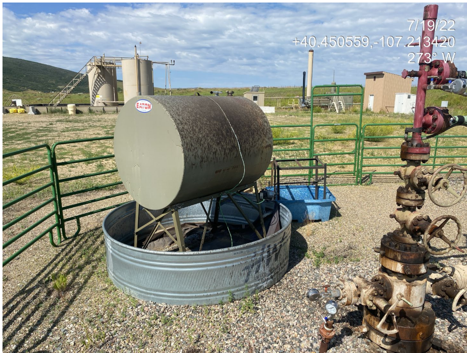
Photo 12. Photo shows a methanol tank adjacent to the well with missing/insufficient wildlife protection BMPs on the secondary containment stock tank.
