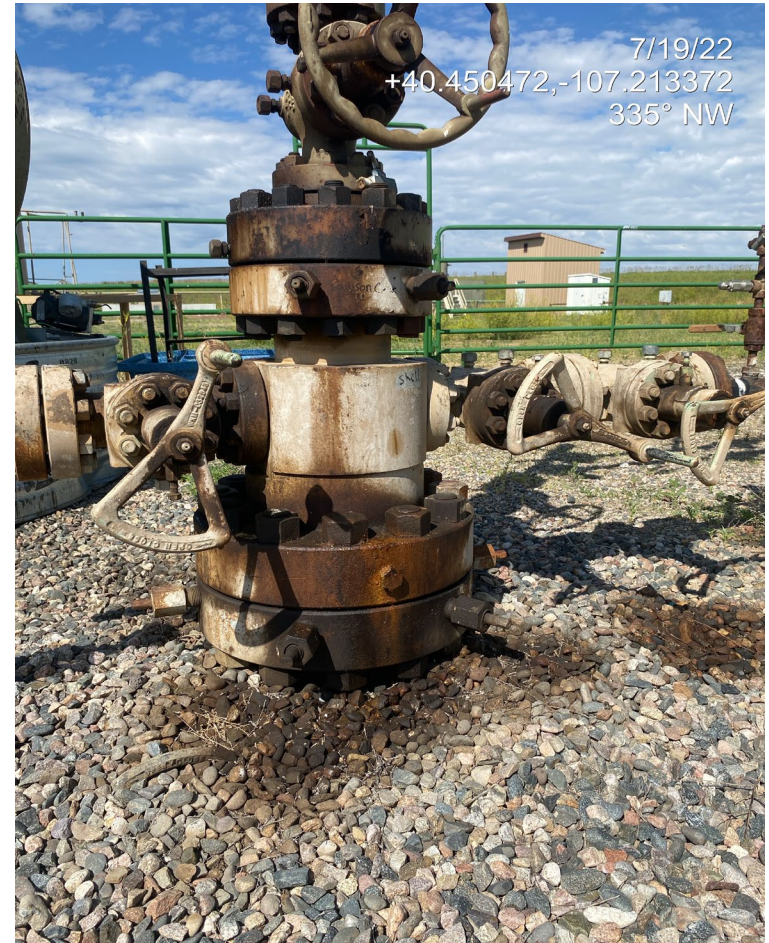
Photo 11. Photo taken from the well area shows impacted soils around the wellhead.
