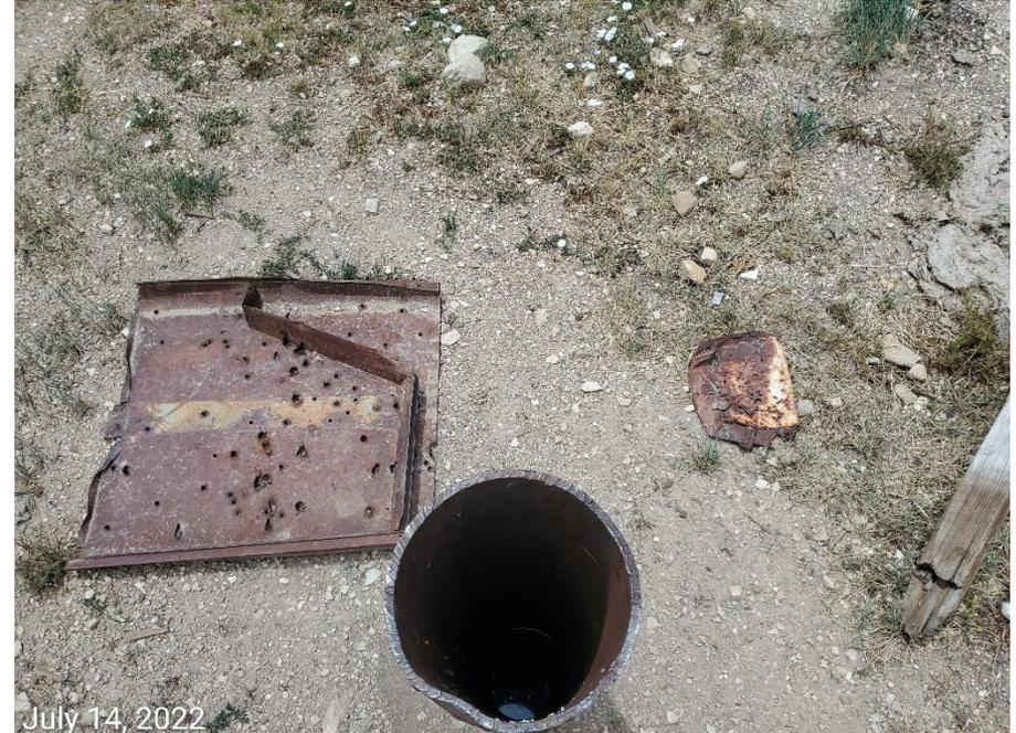
**Photo 1:** Photos shows well marker has not been installed per (pre-1/15/2021 rule change) Rule 319.a.(5). Pipe has missing welded plate at top, and is currently open.
