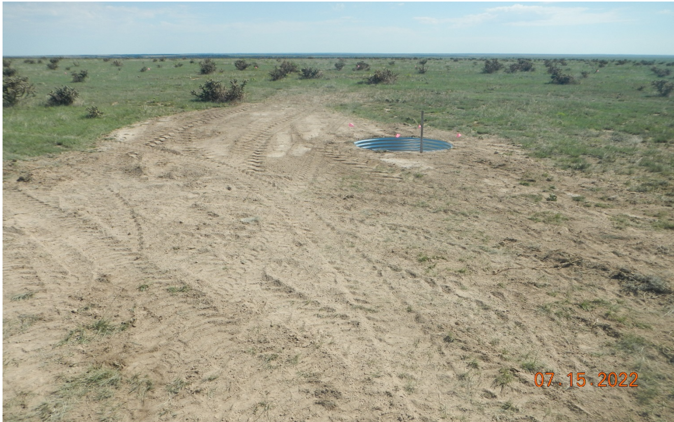
Photo 4. Facing northeast. A conductor has been set in preparation of drilling. The open culvert needs to be covered up to prevent wildlife or livestock entry.
