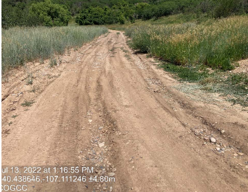
Lack of stabilization/compaction/erosion
