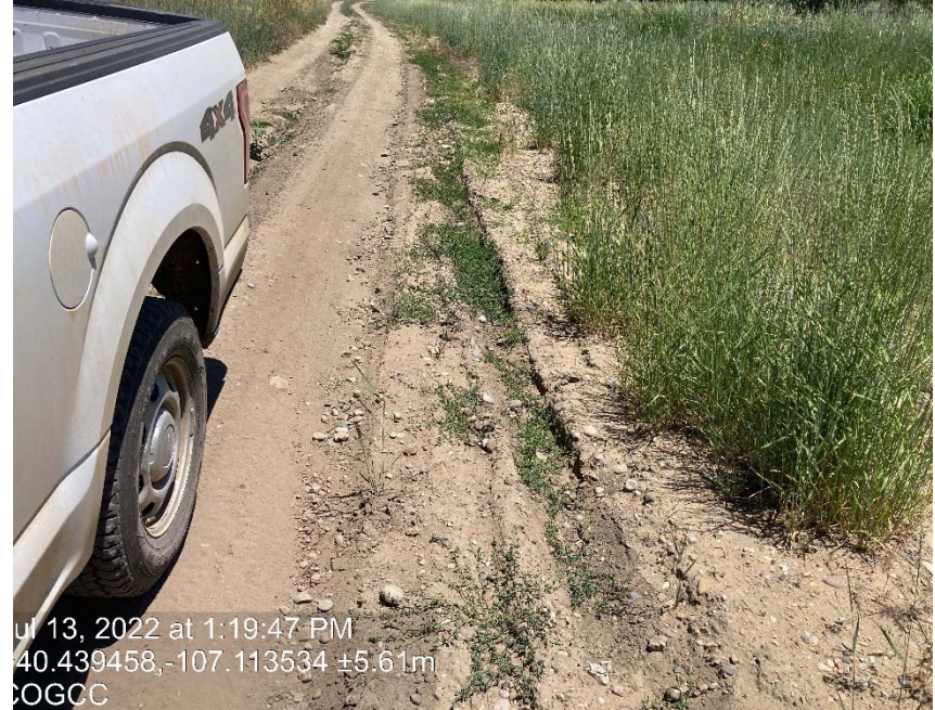
Lack of stabilization/compaction/erosion
