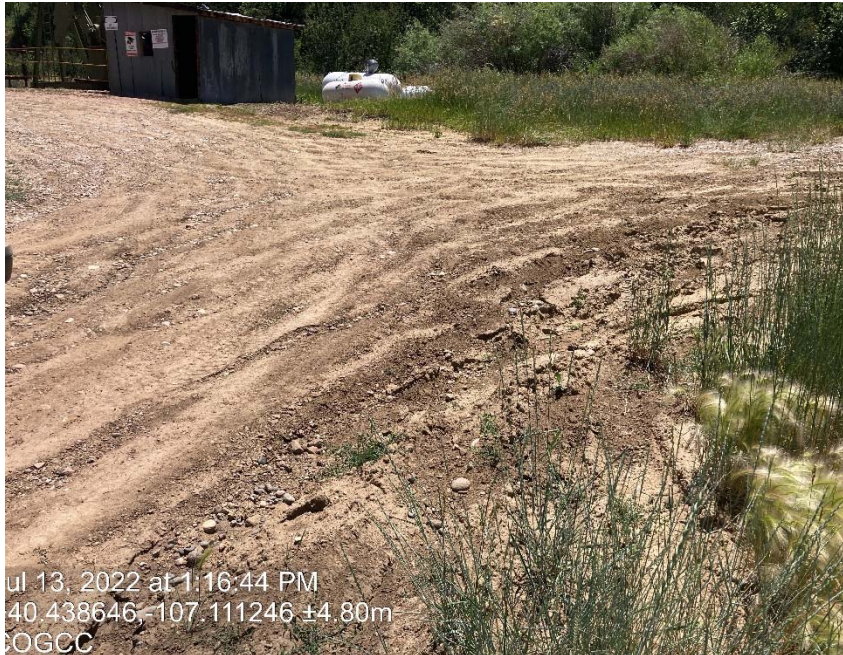
Lack of stabilization/compaction/erosion
