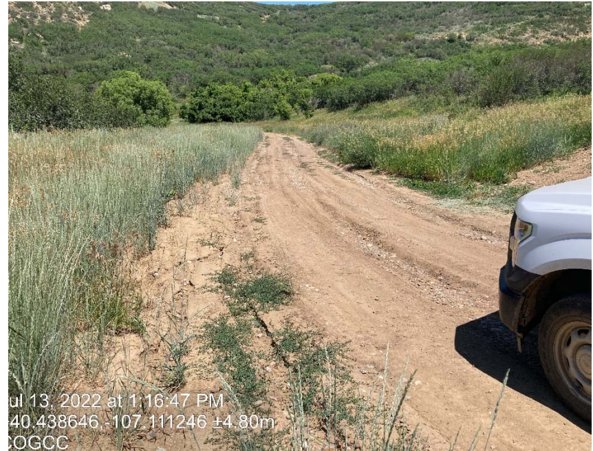
Lack of stabilization/compaction/erosion
