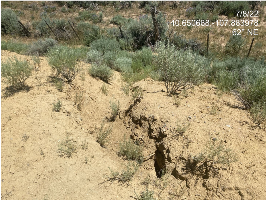
Photo 5. Photo taken from the south of the Location shows gully erosion occurring on sparsely vegetated, unstabilized slopes of the Location.
