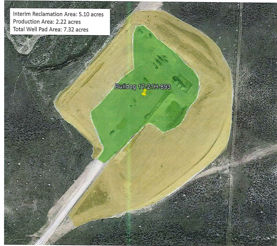
Photo 4. Photo shows the “Location Drawing” from document #401412049 which shows an estimate of production areas and interim reclamation areas included in variance request document #401291906. Variance expired 5/1/2022. Interim reclamation is required.
