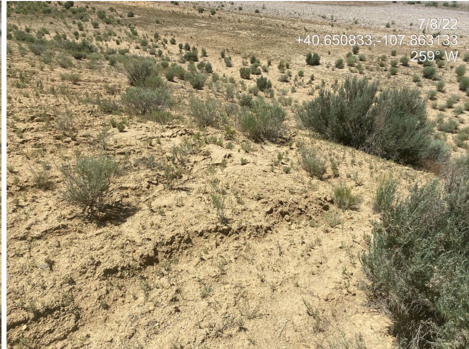
Photo 8. Photo taken from the east of the Location shows gully erosion occurring on sparsely vegetated, unstabilized slopes.
