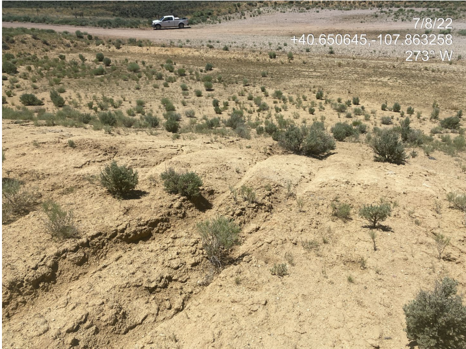
Photo 7. Photo taken from the southeast of the Location shows gully erosion occurring on sparsely vegetated, unstabilized slopes.
