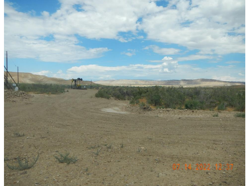
Ditch on access road has been maintained.
