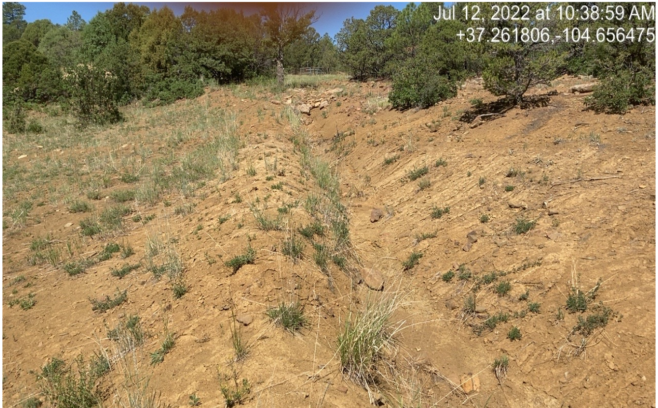
Photo 6. Facing toward the northwest side of the location. This area will need additional stabilization and BMP's to prevent erosion.
