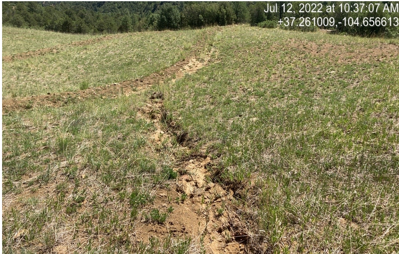
Photo 4. There is an erosion channel at the south side of the offsite pit which will need BMP's to prevent further erosion.
