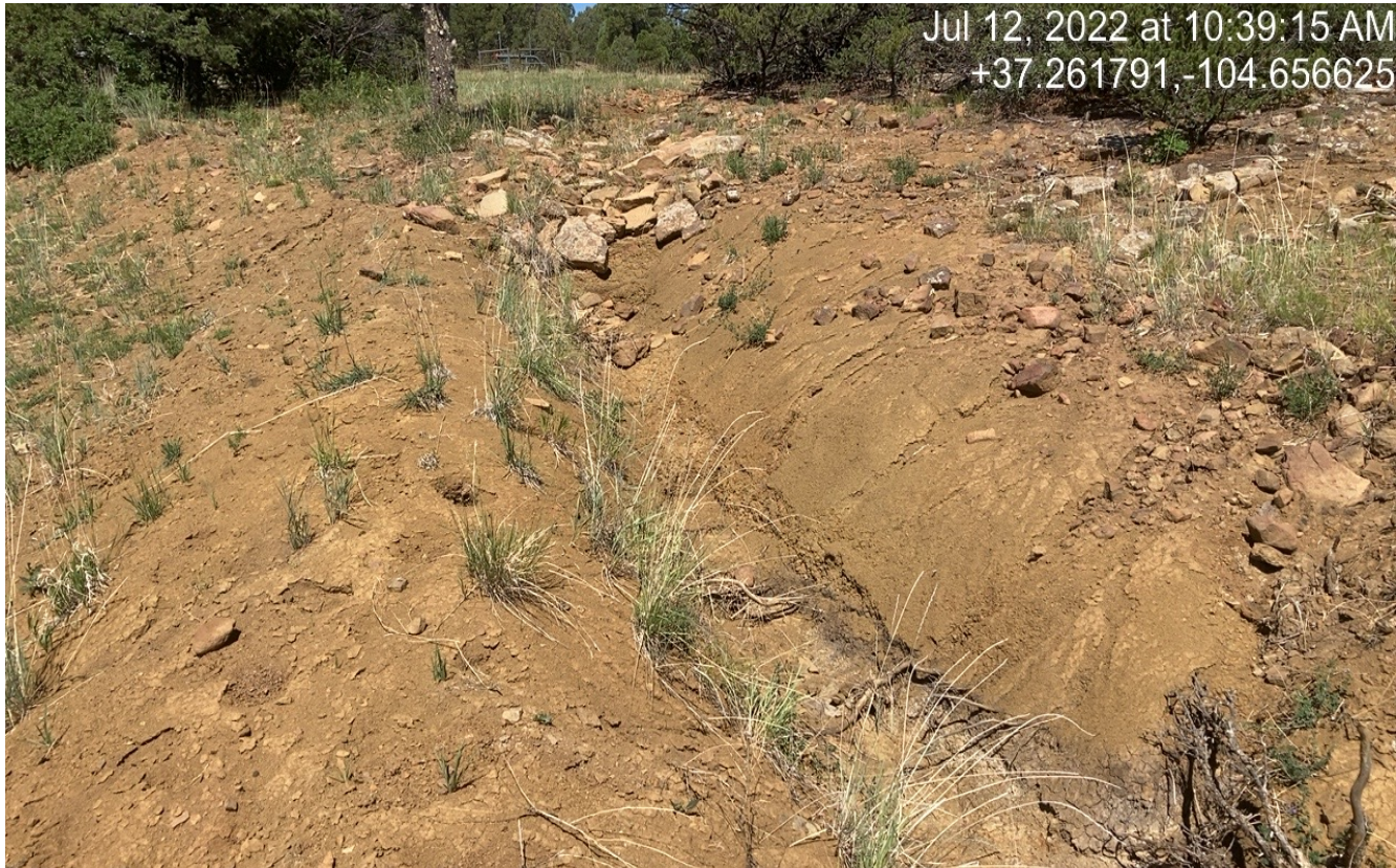
Photo 7. This area will need additional stabilization and BMP's to prevent erosion. Stormwater is directed toward this area from the main road.
