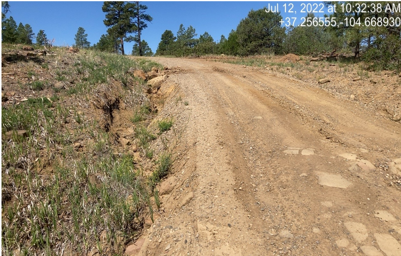
Photo 2. Facing west along the main access road. There is erosion along the roadside in this area.
