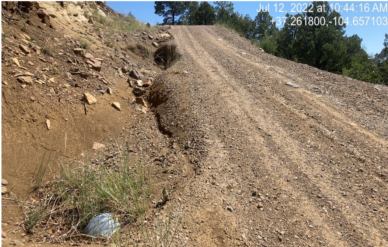
Photo 1. Facing northeast along the main access road past the compressor. There is erosion along the roadside in this area and the culvert is partially filled in with sediment.
