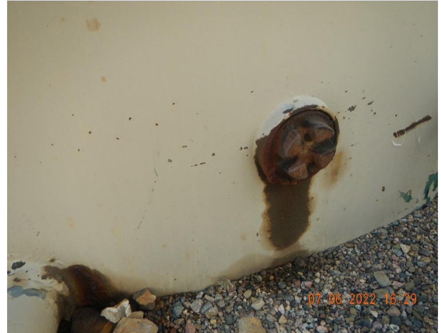
Leaky fittings on bottom of tank.
