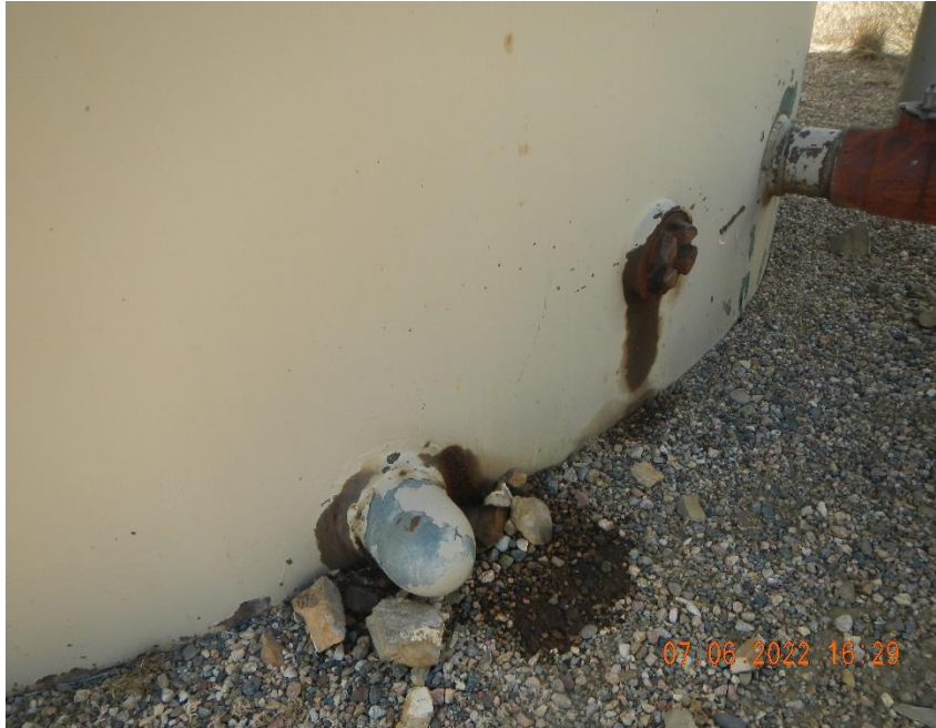
Leaky fittings on bottom of tank.
