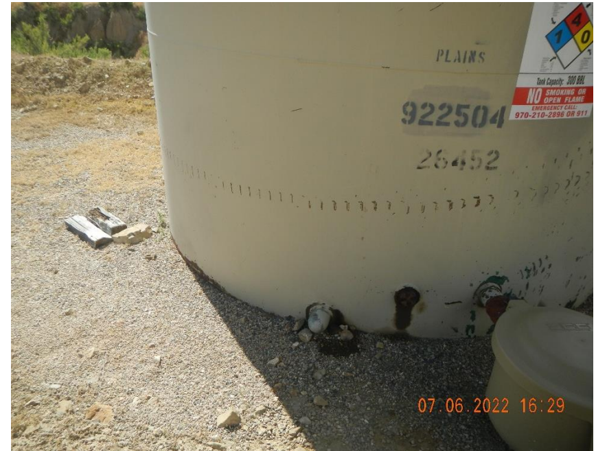
Leaks from tank fittings.
