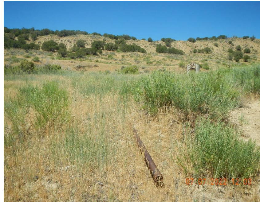
Open ended unused flow line running off location.
