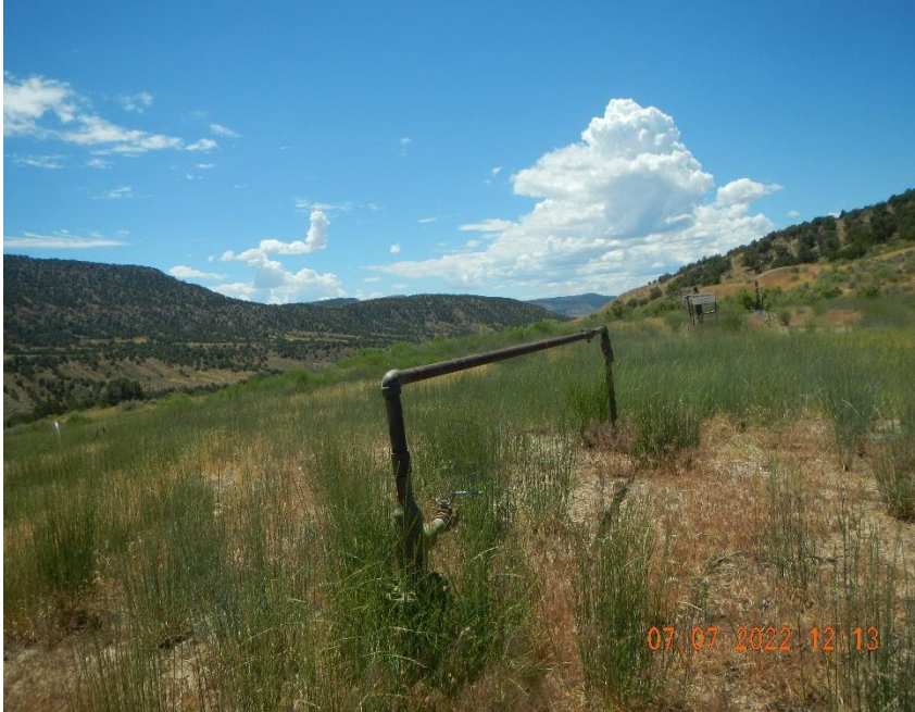
3" open ended riser in front of flow line.
