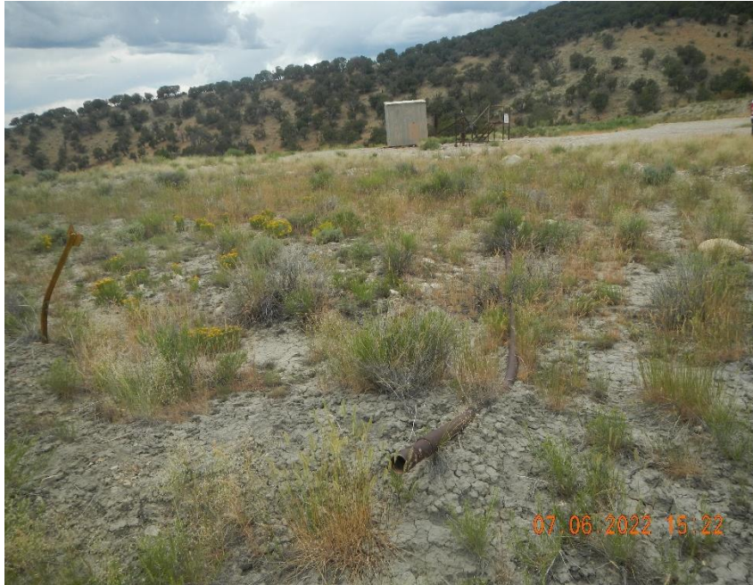
Unused flow lines on location.
