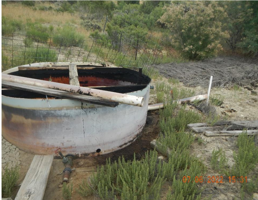
Hydrocarbon build up in pit and in tank at intake line from well.
