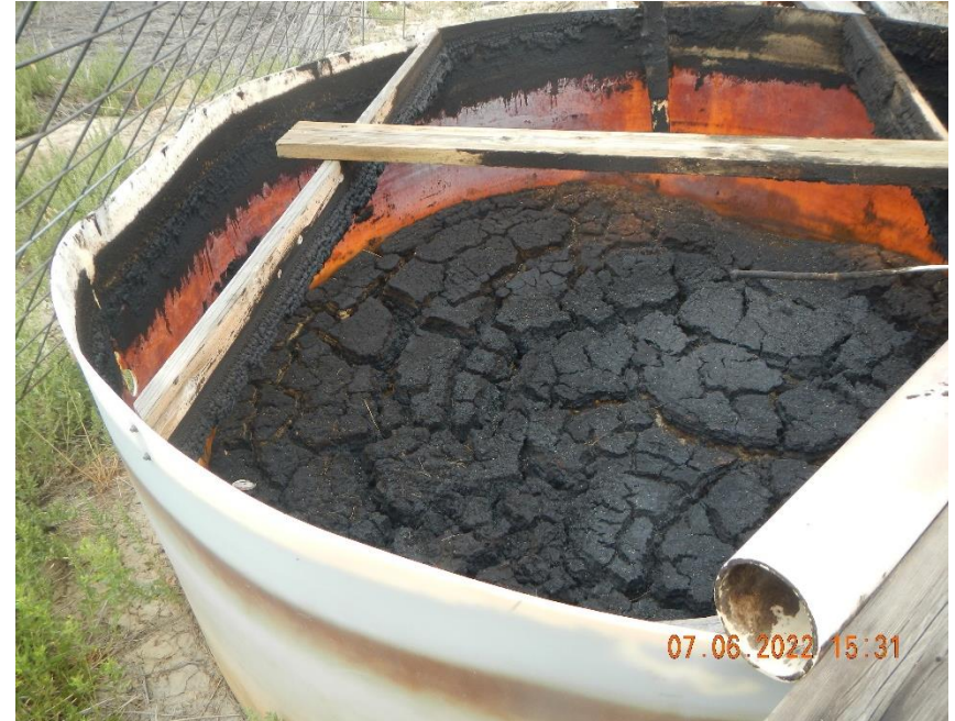
Hydrocarbon build up in pit and in tank at intake line from well.
