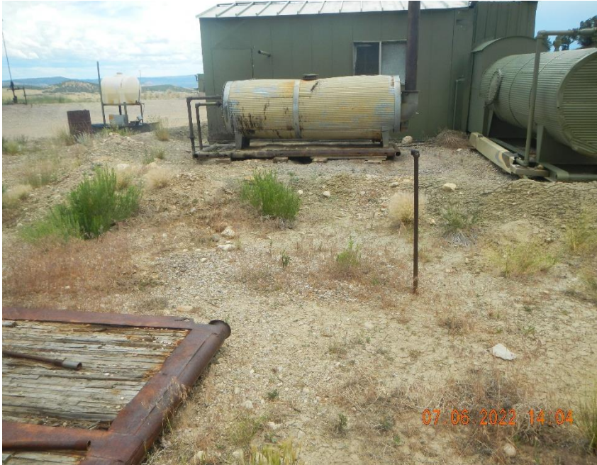
Open ended 1" riser at separation equipment.
