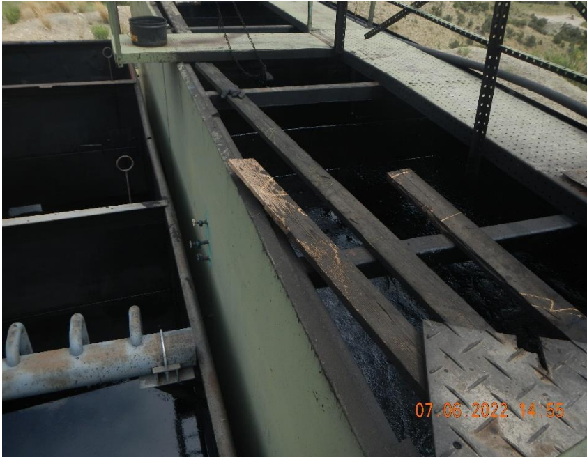
Crude oil in open top tank. No netting for wildlife protection.
