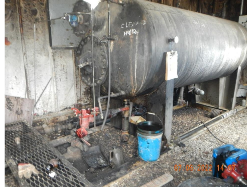
Buckets of oil with no lids not stored in secondary containment in side of separator shed.
