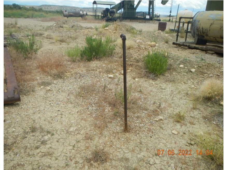
Open ended 1" riser at separation equipment.
