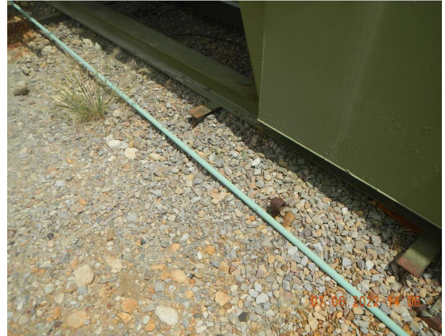
Open ended 1" riser at separation equipment.
