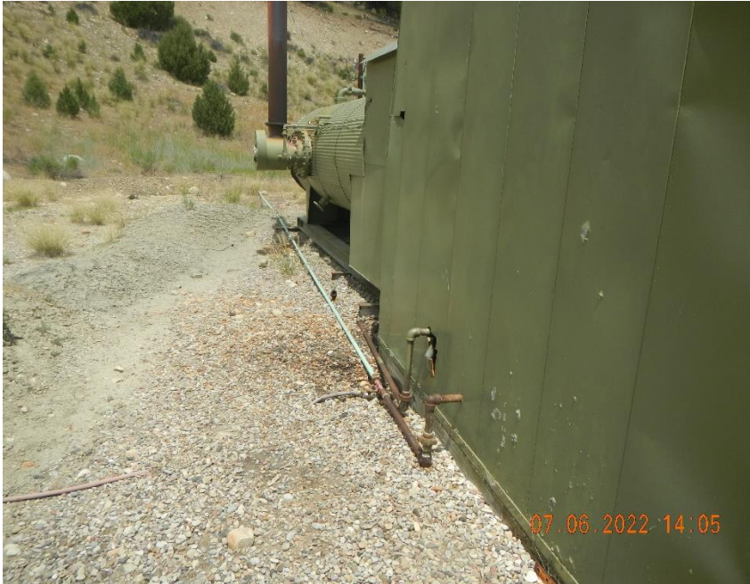
Open ended 1" riser at separation equipment.
