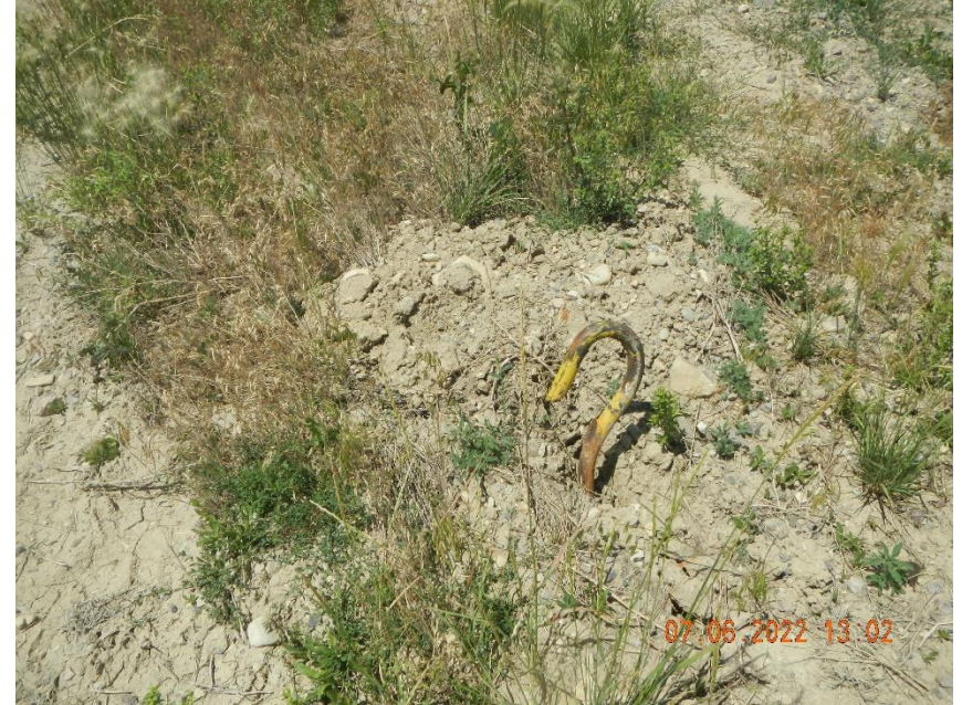
Unmarked and damaged deadman in center of location.
