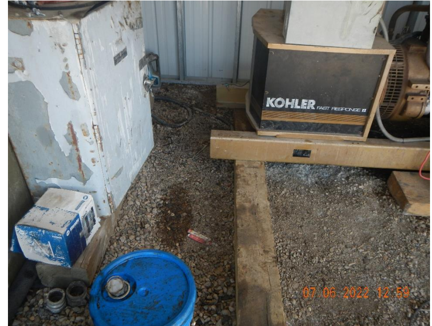
Motor and lube oil staining ground under and around injection engine and pump.
