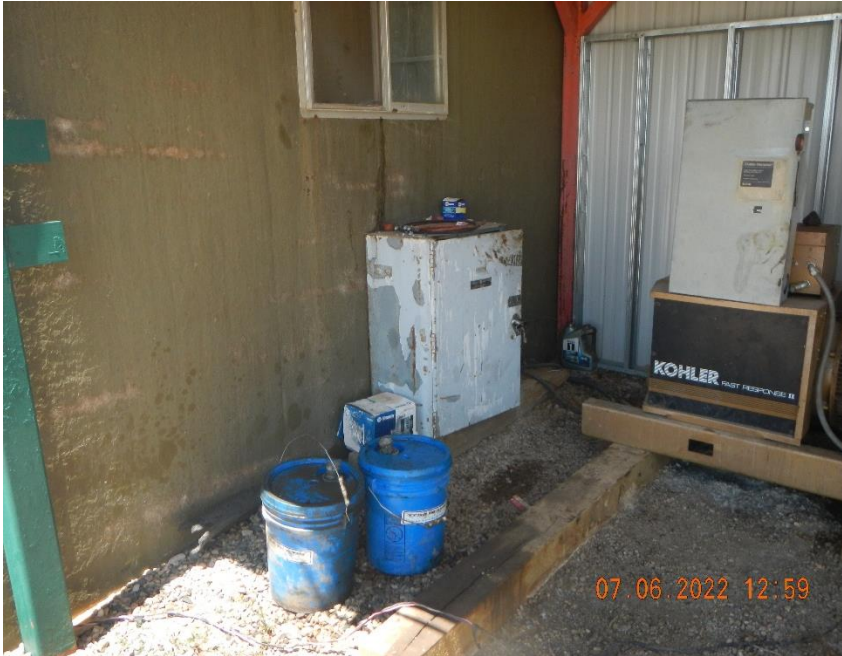
Motor oil buckets no secondary containment.
