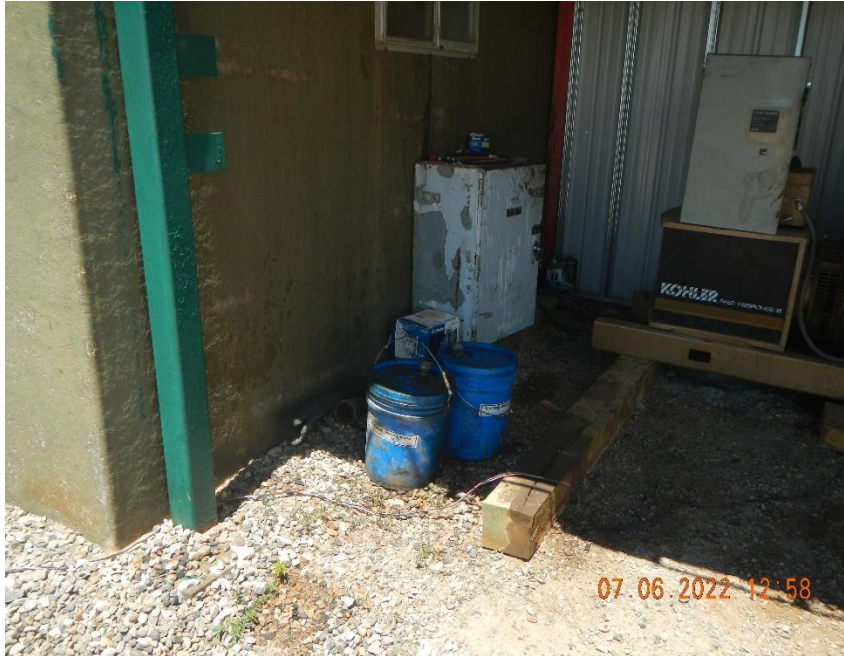
Motor oil buckets no secondary containment.
