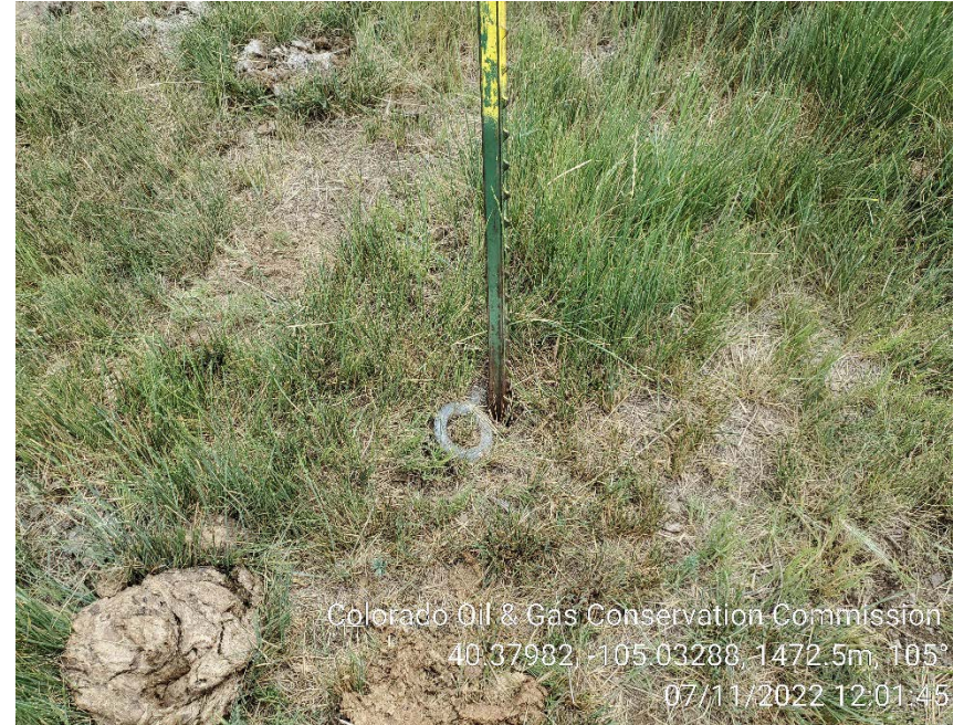
Guy line anchor on 7/11/2022
