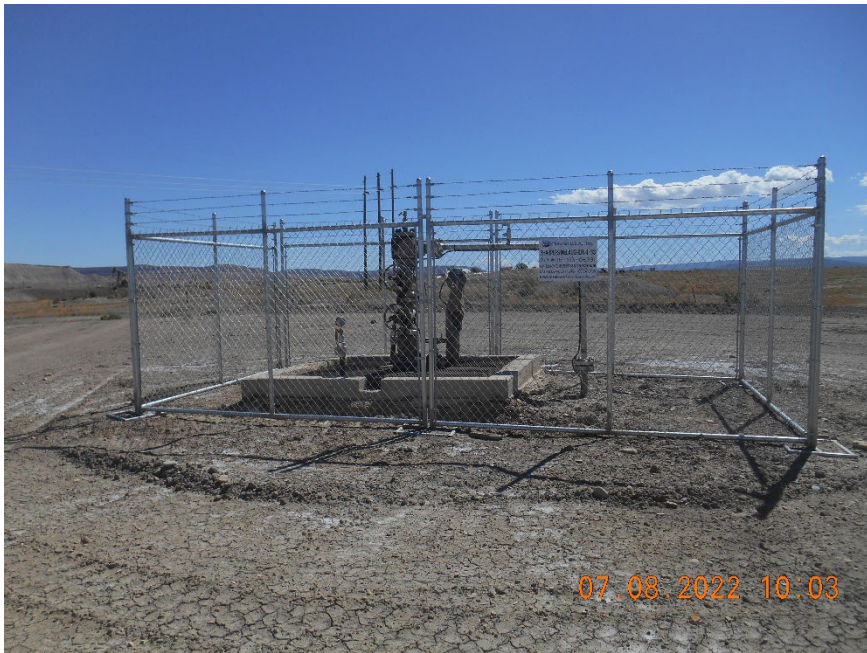
Injection wellhead
