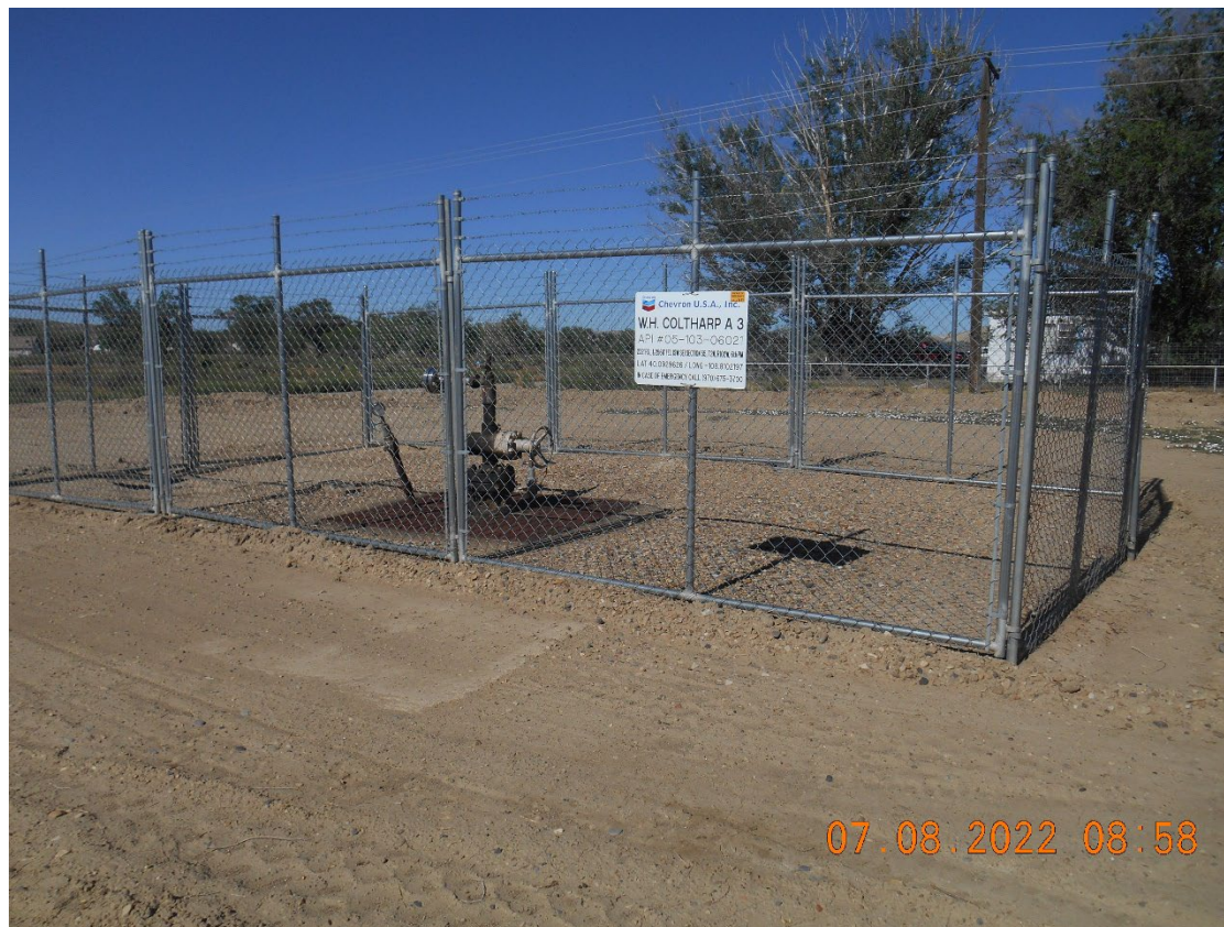
Injection wellhead. Temporarily Abandoned
