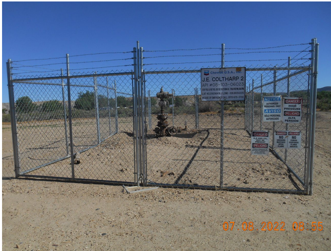
Injection Wellhead – Temporarily Abandoned
