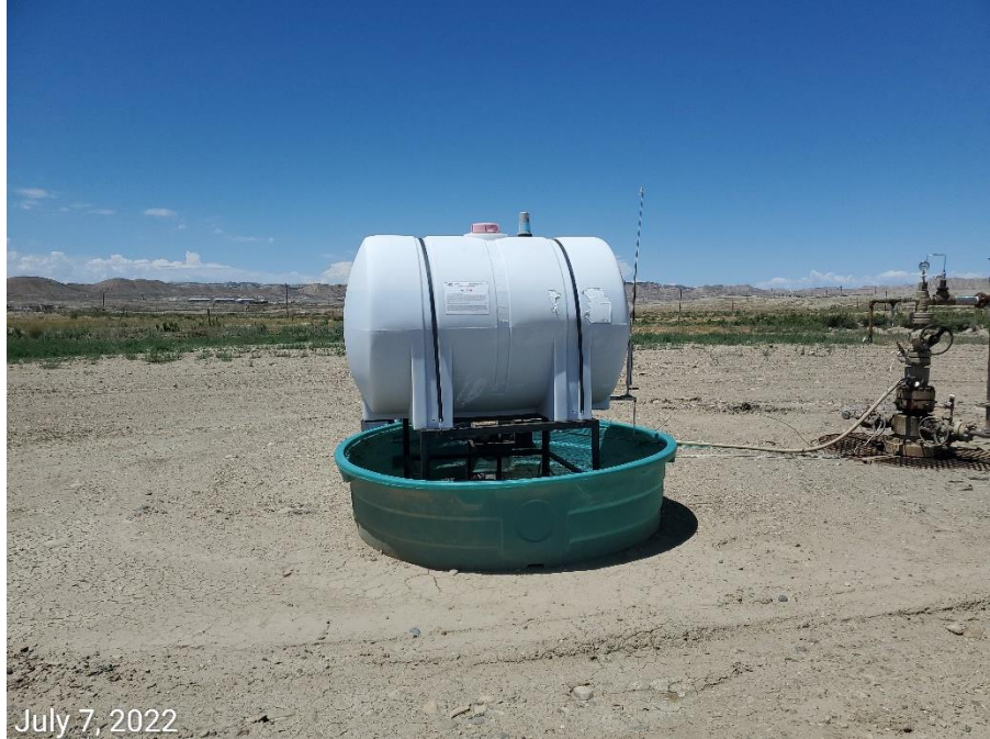
Photo 1: Photo show fluids within containment at the methanol tank.
