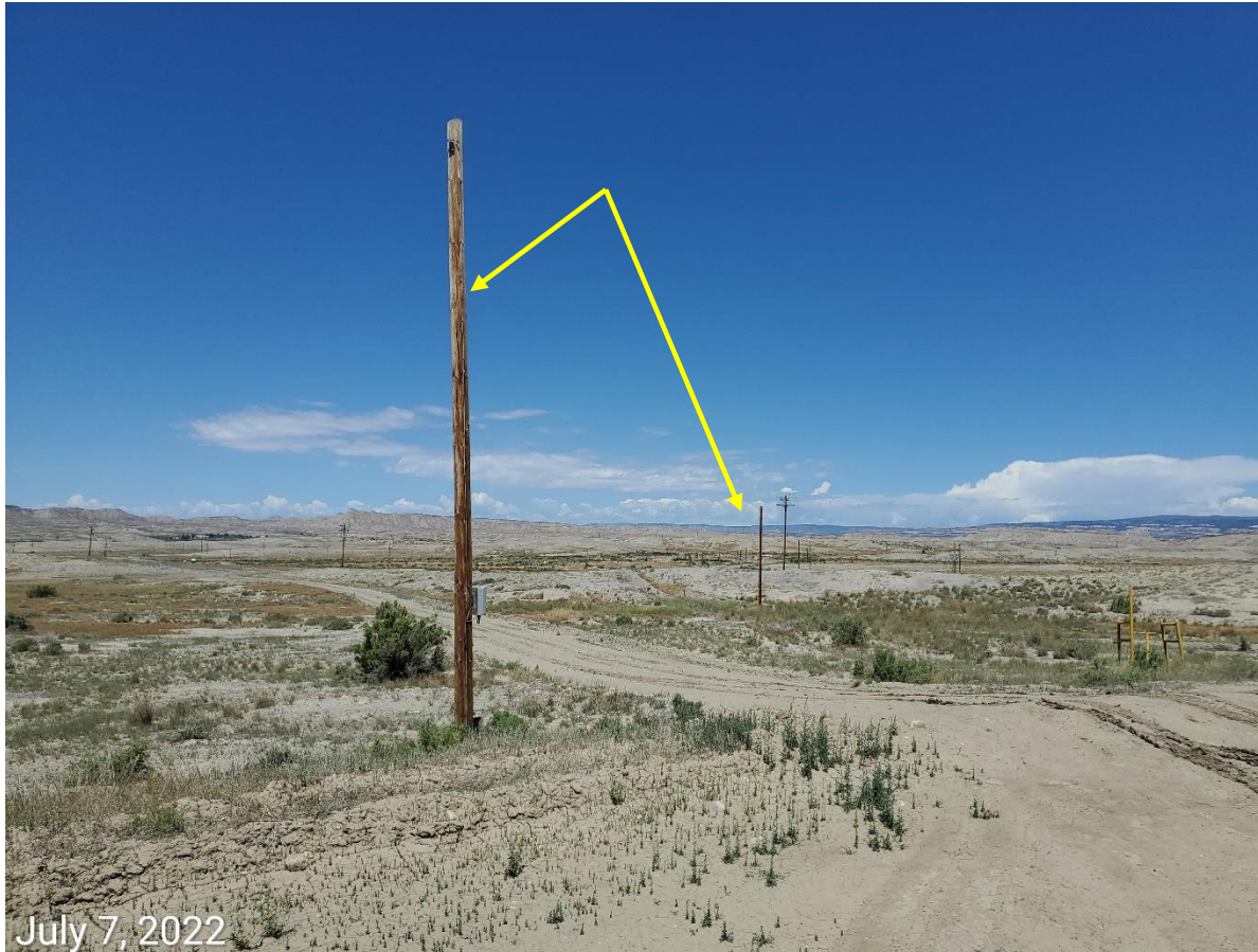
Photo 5: Photo shows unused utility pole equipment leading two the Location; lines have been removed and poles have been left behind
