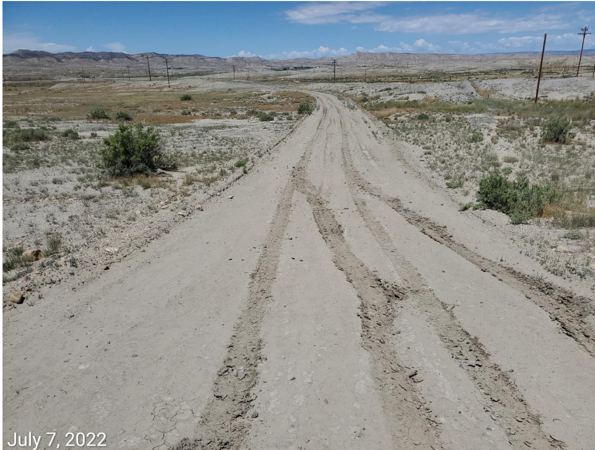
Photo 4: Photo example showing stabilization issues resulting in vehicle tracking and sediment transport on the access road(s).
