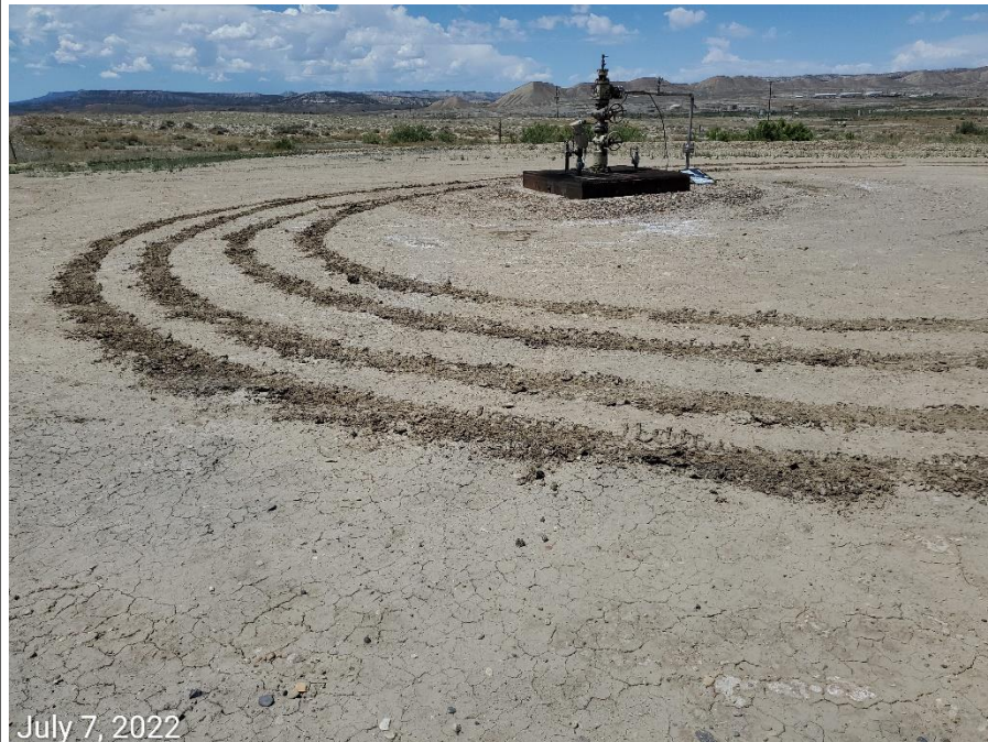
Photo 3: Photo shows vehicle tracking/rutting evident on the pad. Control measures to minimize degradation and sediment transport are missing or insufficient at the Location, and the two access roads leading south and west from the Location
