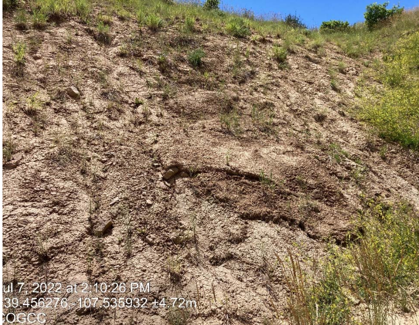
Lack of stabilization/ erosion
