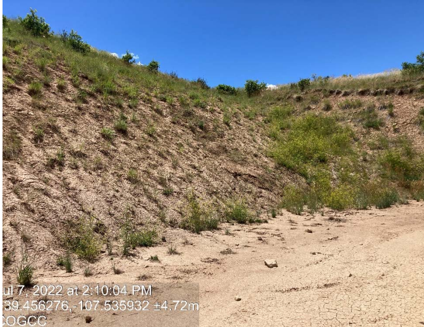
Lack of stabilization/ erosion
