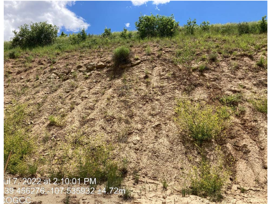
Lack of stabilization/ erosion
