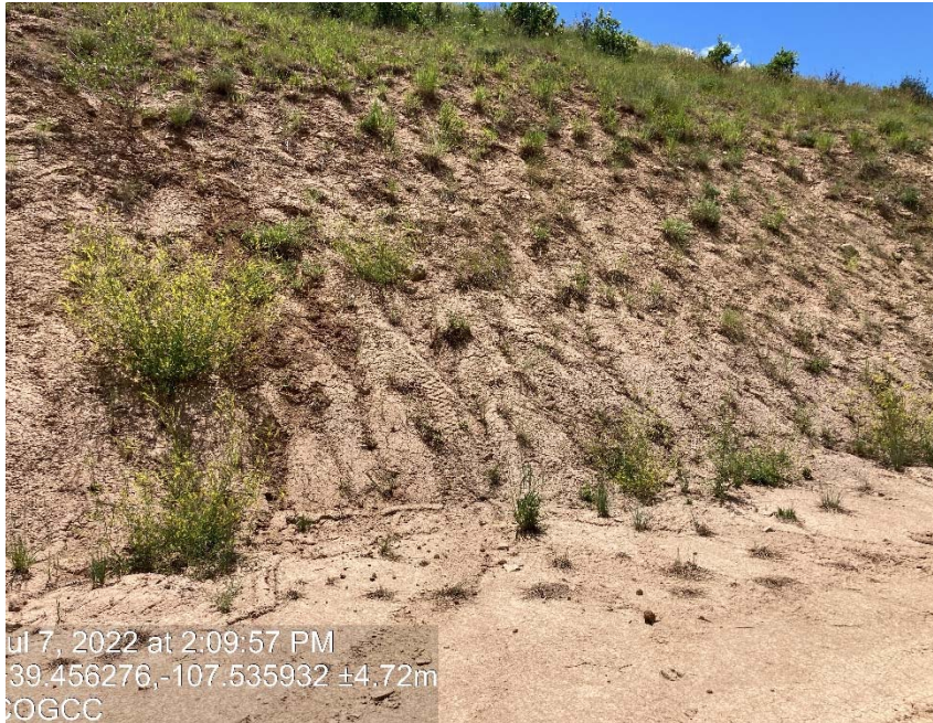
Lack of stabilization/ erosion
