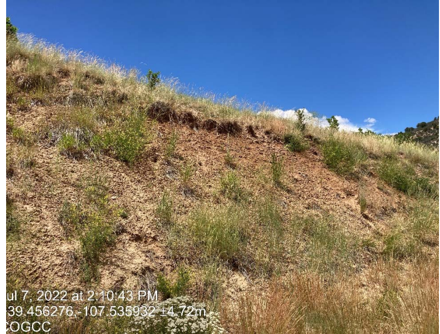
Lack of stabilization/ erosion
