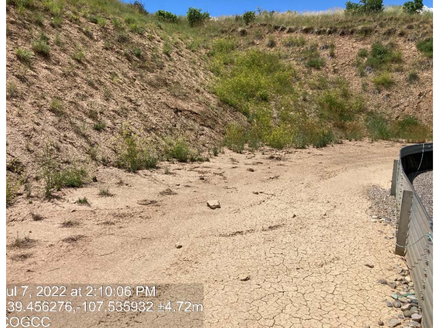
Lack of stabilization/ erosion
