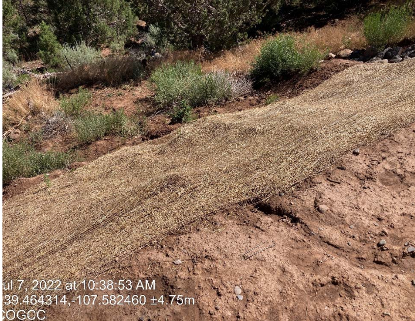
Rill erosion under erosion blanket
