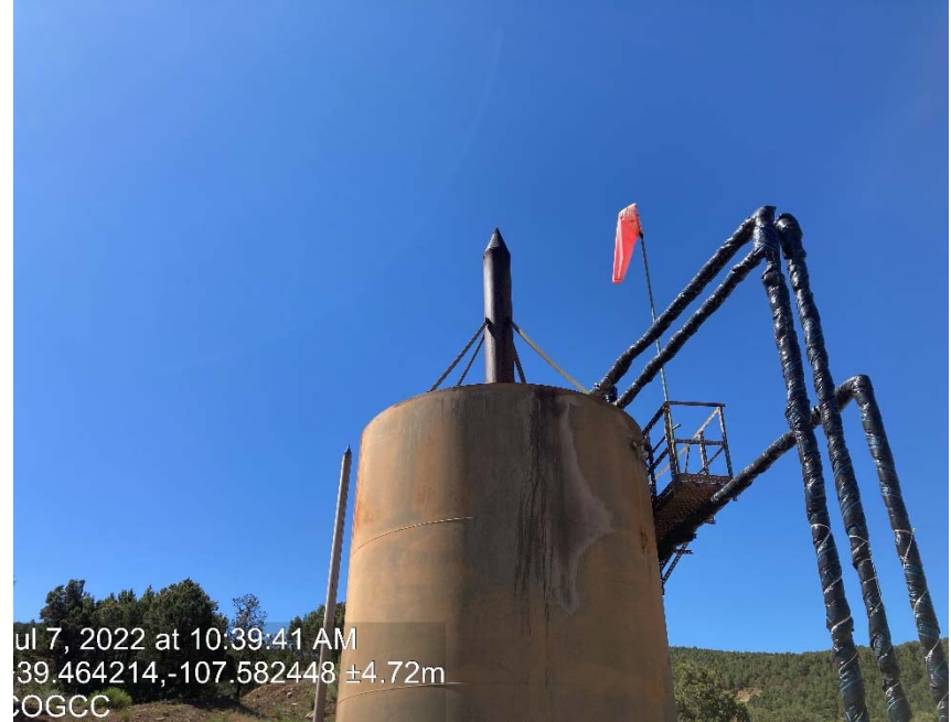
Open vent on condensate tank
