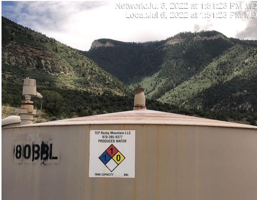
Photo #7079 Vent pipe on tank open ended.
