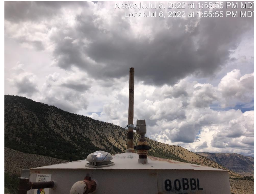
Photo #7083 Vent pipe open ended.
