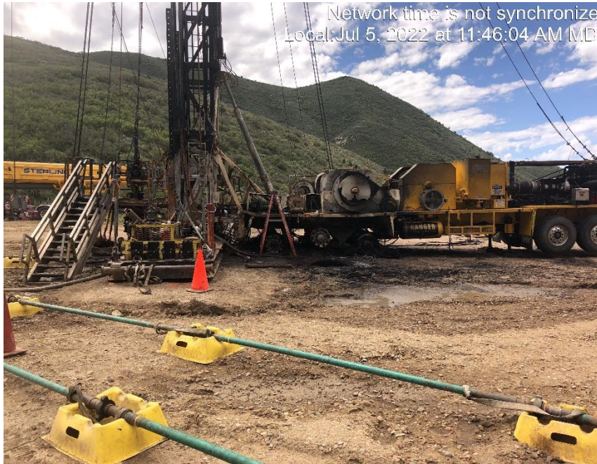
Photo #7067 Turbo side of workover rig.
