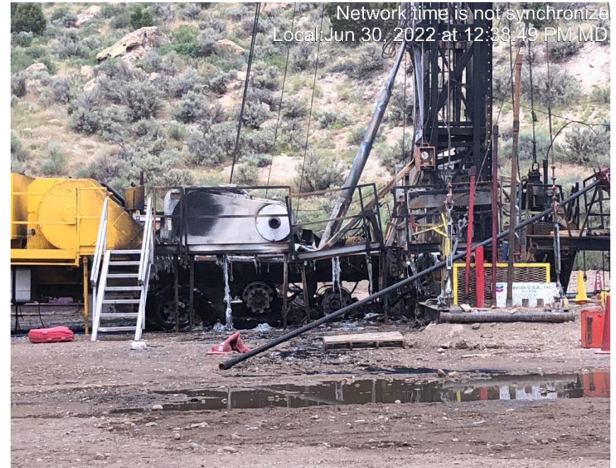
Photo #7054 cab side of workover rig fire from inspection #699804662 conducted on 6/30/22.
