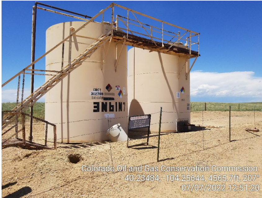
Photo 1 – Tank Battery
