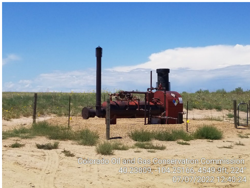
Photo 3 – Separator and ECD
