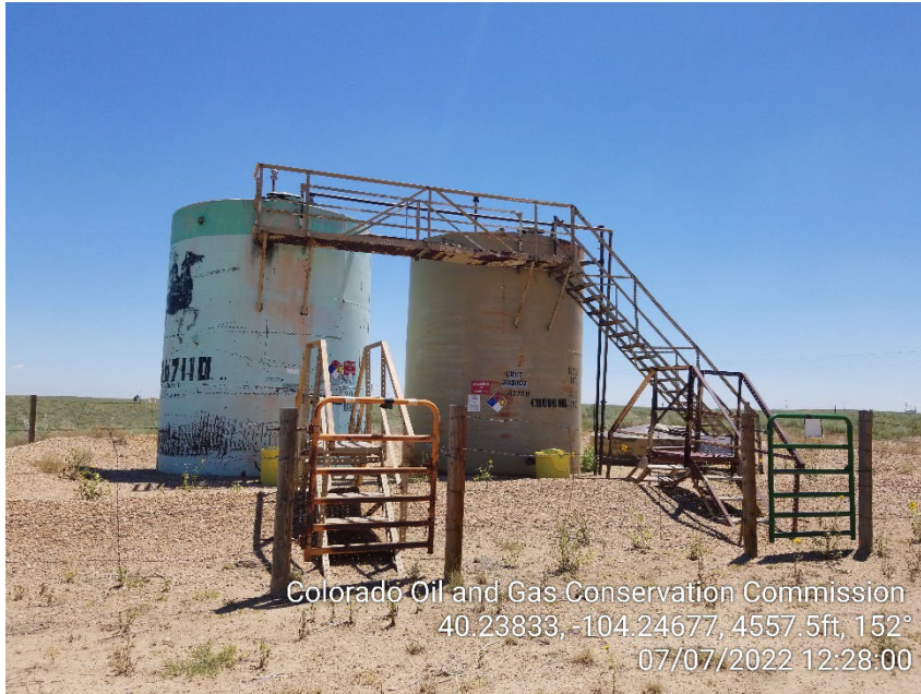
Photo 1 – Tank Battery
