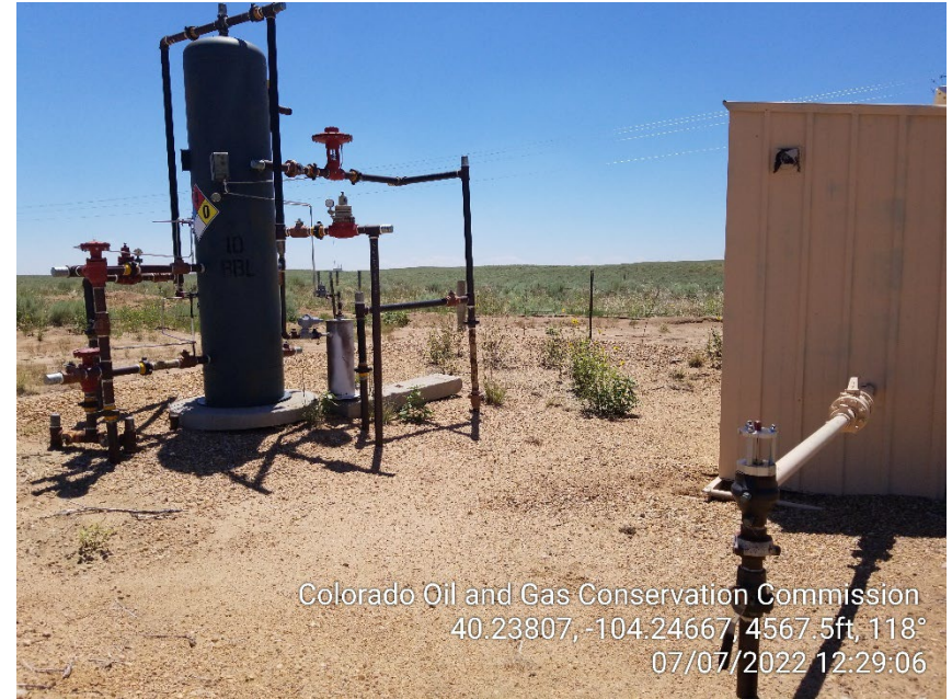
Photo 4 – Separator and Gas Meter
