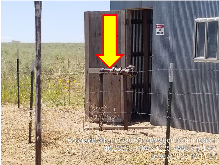
Photo 5 – Unmarked Risers
