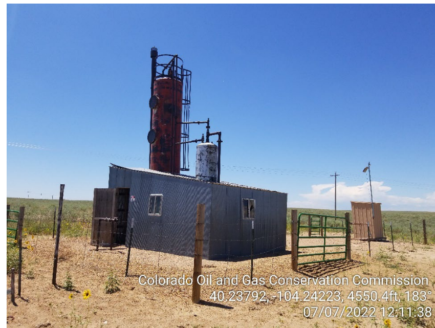
Photo 4 – Heater Treater
