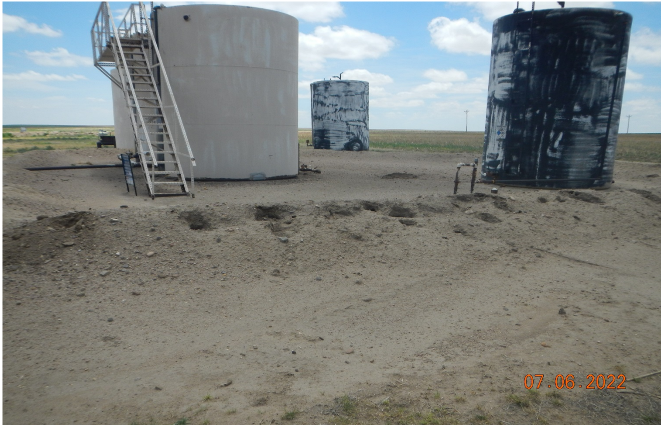
Photo 2. The berm around the tank battery is inadequate with animal boroughs.
