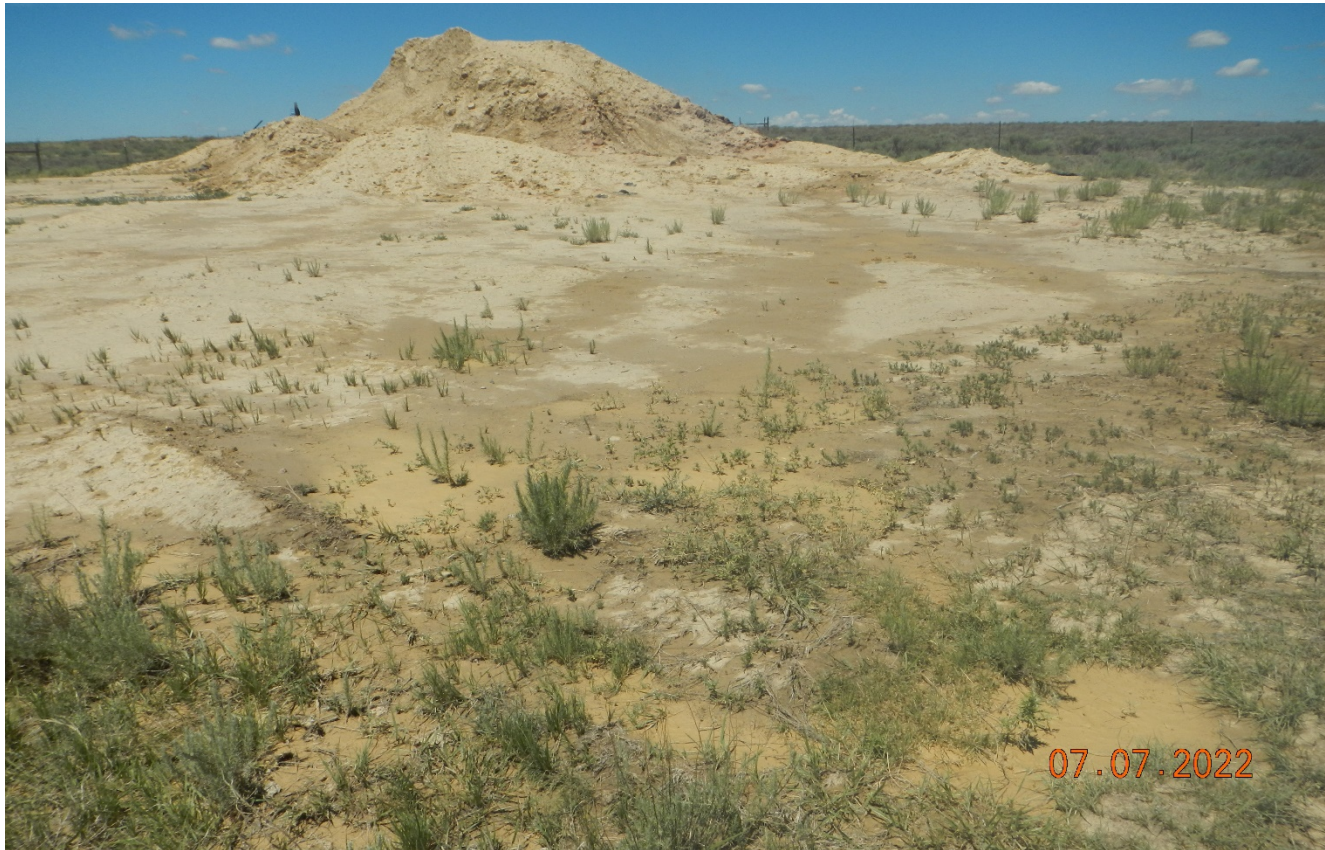
Photo 11. Facing west toward the excavated material stored onsite. There are no perimeter BMP's around the excavated material to prevent sediment transport offsite. There are signs this material has eroded offsite from recent precipitation.
