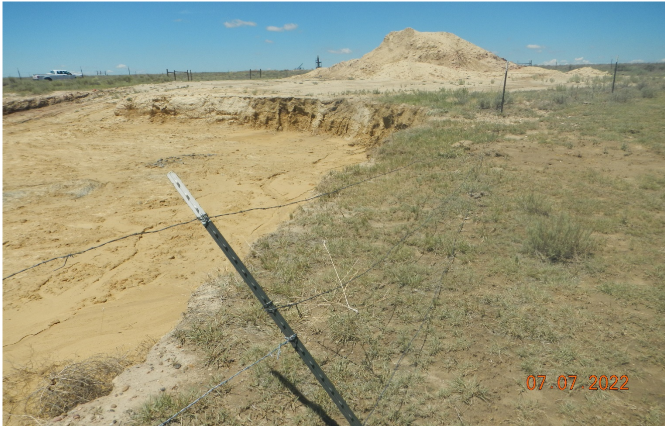
Photo 10. Facing west toward the excavated area. The fence around the location is inadequate to prevent livestock entry and is not maintained.
