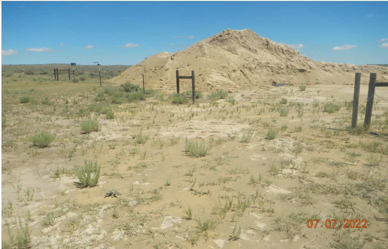
Photo 6. Facing north toward the location. There is a remediation project # 19874 in process with excavated material stored onsite. There are no perimeter BMP's around the excavated material to prevent sediment transport offsite.
