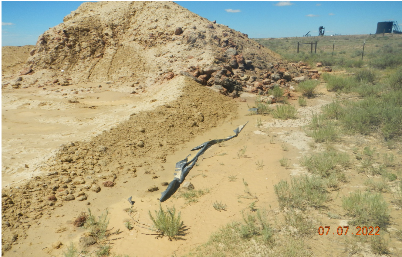
Photo 12. Facing west toward the excavated material stored onsite. There are no perimeter BMP's around the excavated material to prevent sediment transport offsite. There are signs this material has eroded offsite from recent precipitation.
