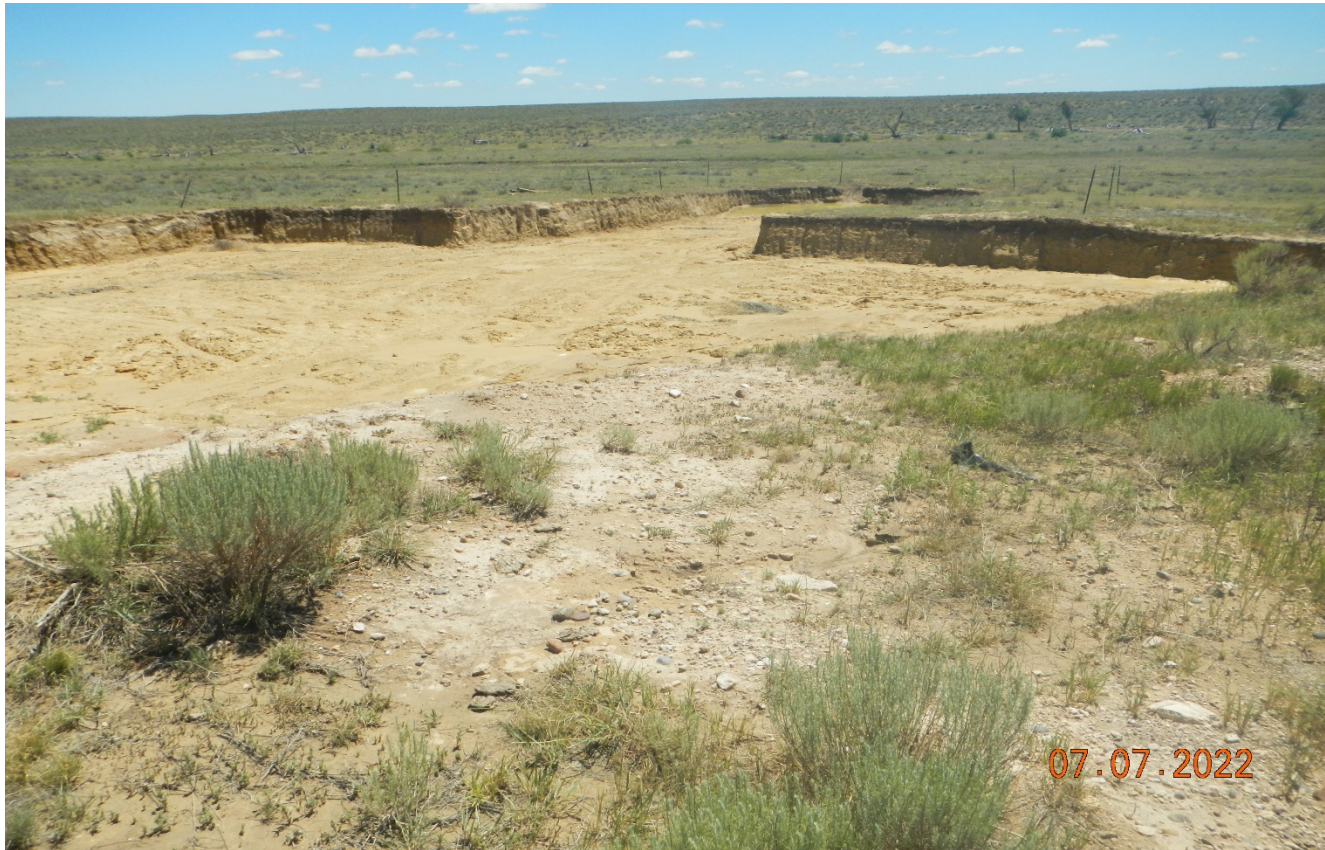
Photo 7. Facing northeast toward the excavated area.
