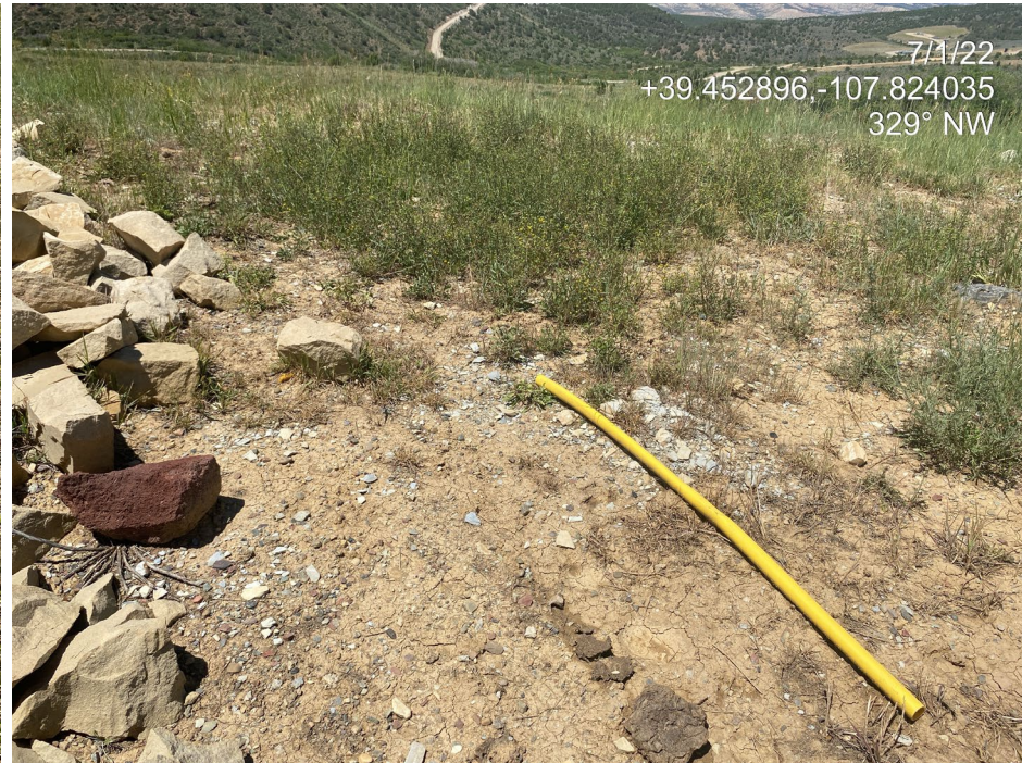
Photo 6. Photo taken at the north of the Location shows an anchor marker in disrepair.
