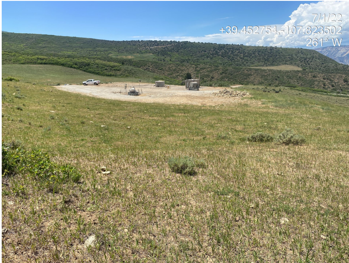
Photo 2. Photo taken from the east of the Location shows interim areas and cut and fill slopes are well vegetated with smooth brome, a non-native perennial grass.
