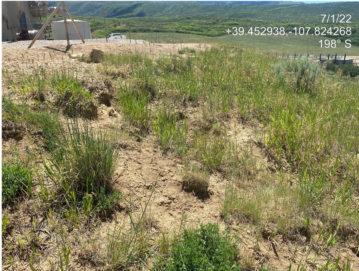
Photo 7. Photo taken from the north of the Location shows erosion degradation to the fill slope.
