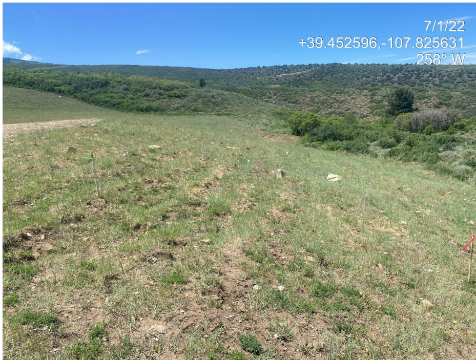
Photo 3. Photo taken from the north shows the fill slope is well vegetated with perennial grasses. Stakes are present indicating areas of partial pad reconstruction.
