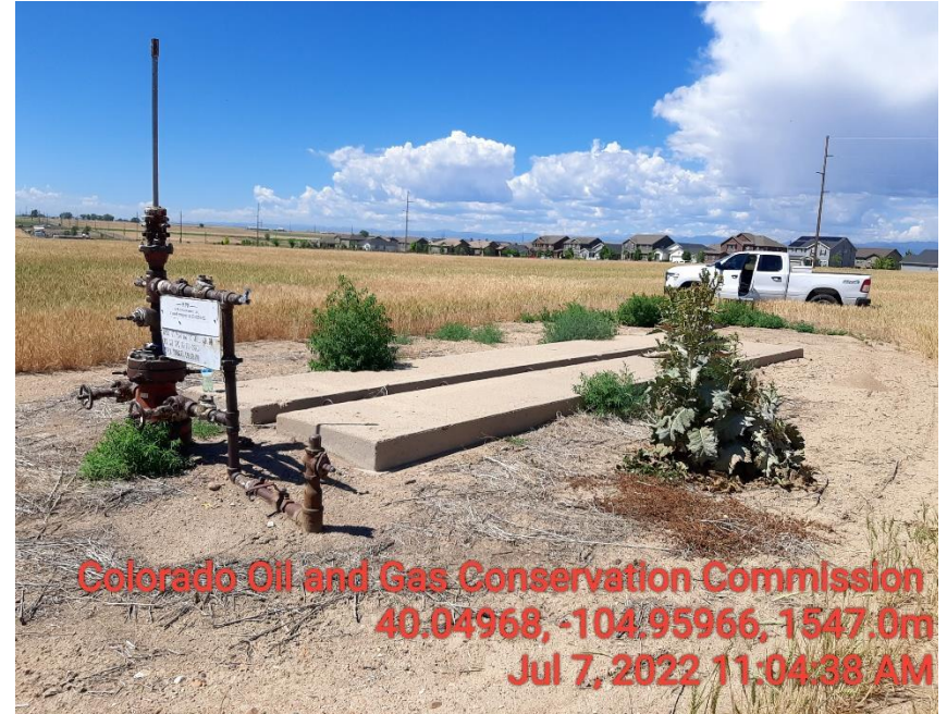
Photo 2 Weeds, unused equipment (cement base) Sign faded not legible.
