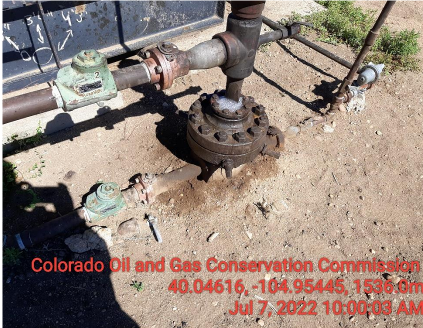
Photo 3 Stained soil and leaking well head around tubing.
