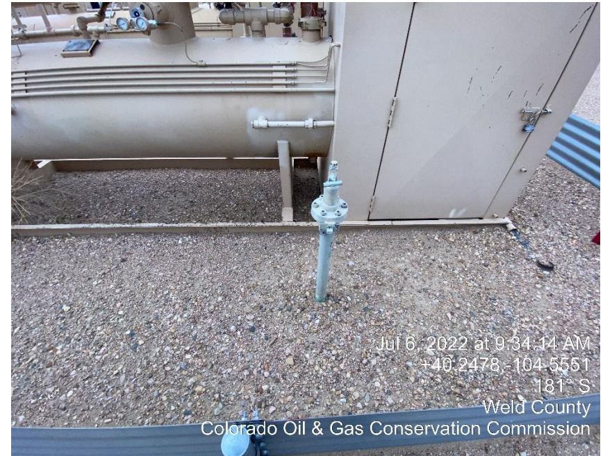
Photo #6 Unmarked Riser
