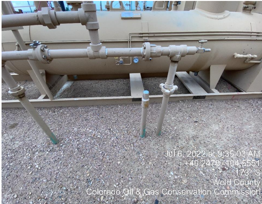
Photo #3 Unmarked Riser
