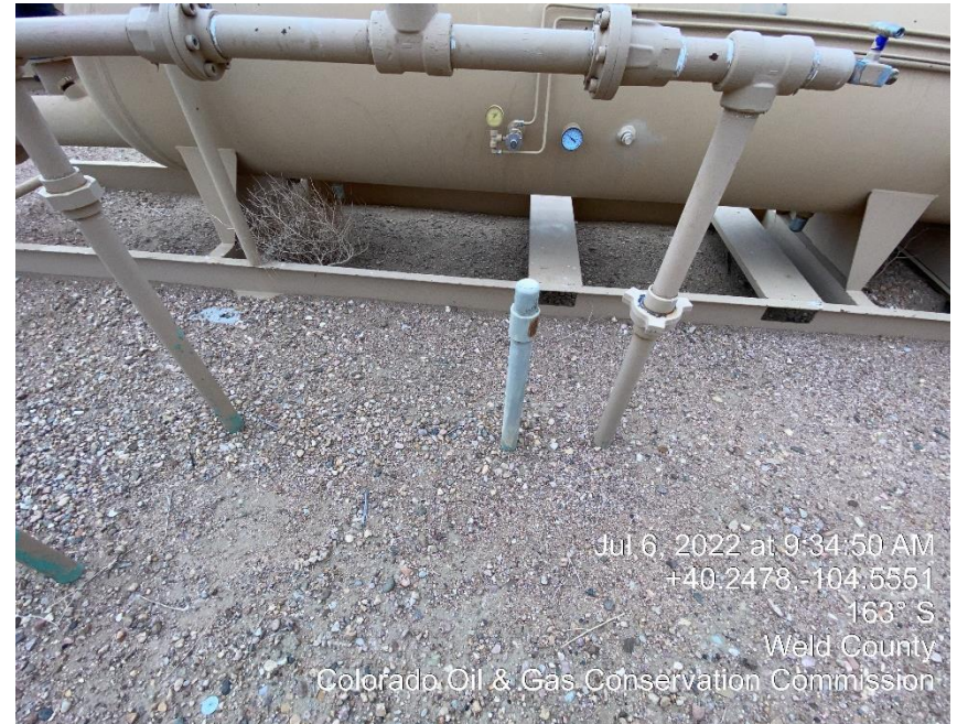
Photo #4 Unmarked Riser
