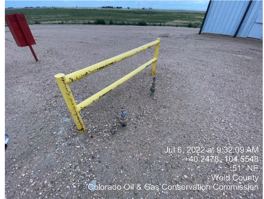
Photo #8 Unmarked Riser
