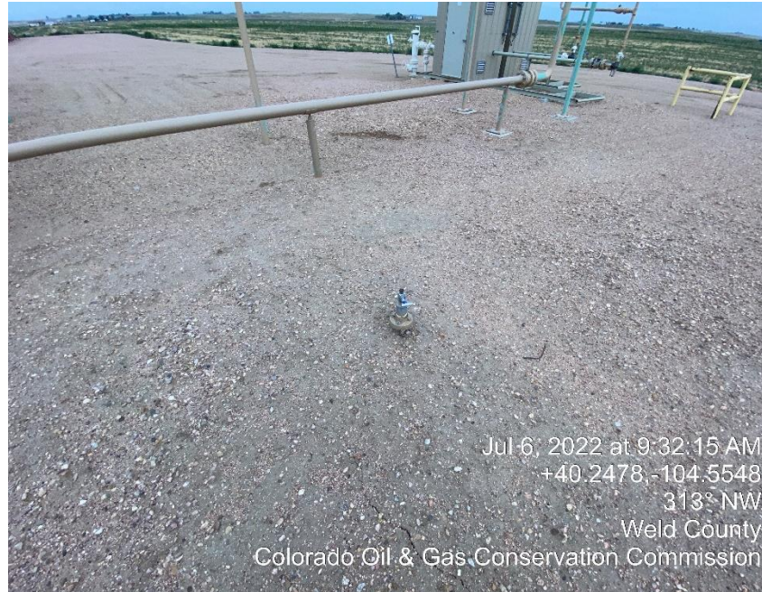
Photo #9 Unmarked Riser
