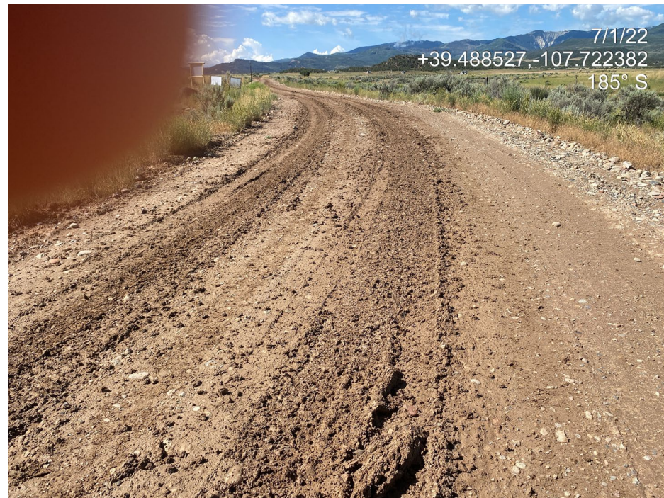
Photo 3. Photo taken from the southwest of the Location shows a lack of stabilization/compaction degradation of the access road.
