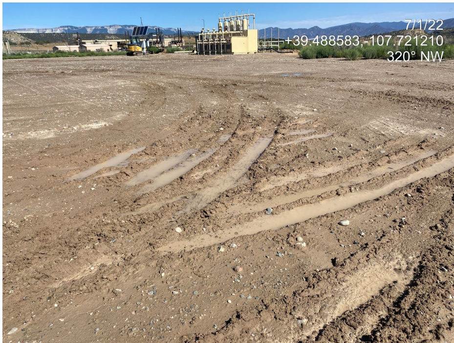
Photo 2. Photo taken from the east of the Location shows a lack of stabilization/compaction degradation of the pad surface.
