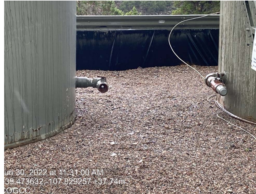
Valve missing cap/plug
