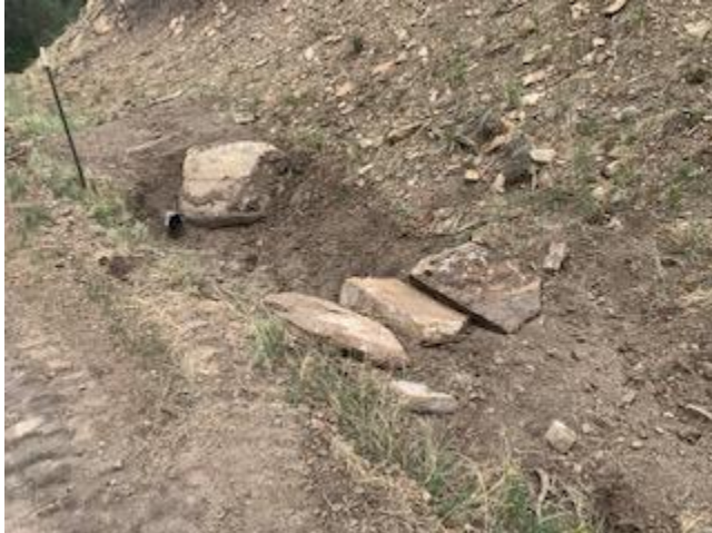
Performed maintenance on Culverts and cleaned out sediment. To comply with Rule 1002.f.(2)C
