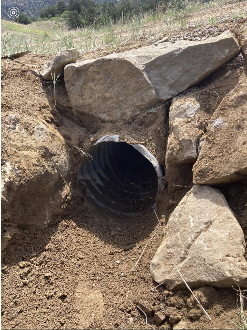
Cleaned out culvert per Rule 1002.f.(2)C
