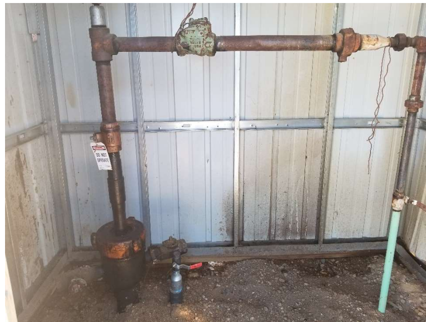
Photo 2. Photo of wellhead inside housing cover. "Do not operate" tag on left.
