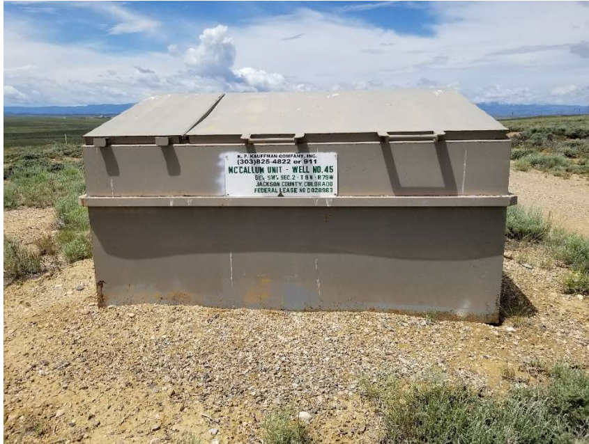
Photo 1. Overview of location taken facing north.
