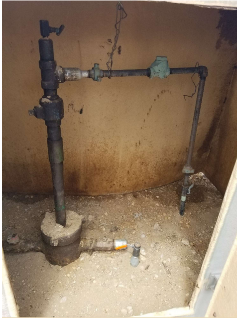
Photo 2. Wellhead inside housing.
