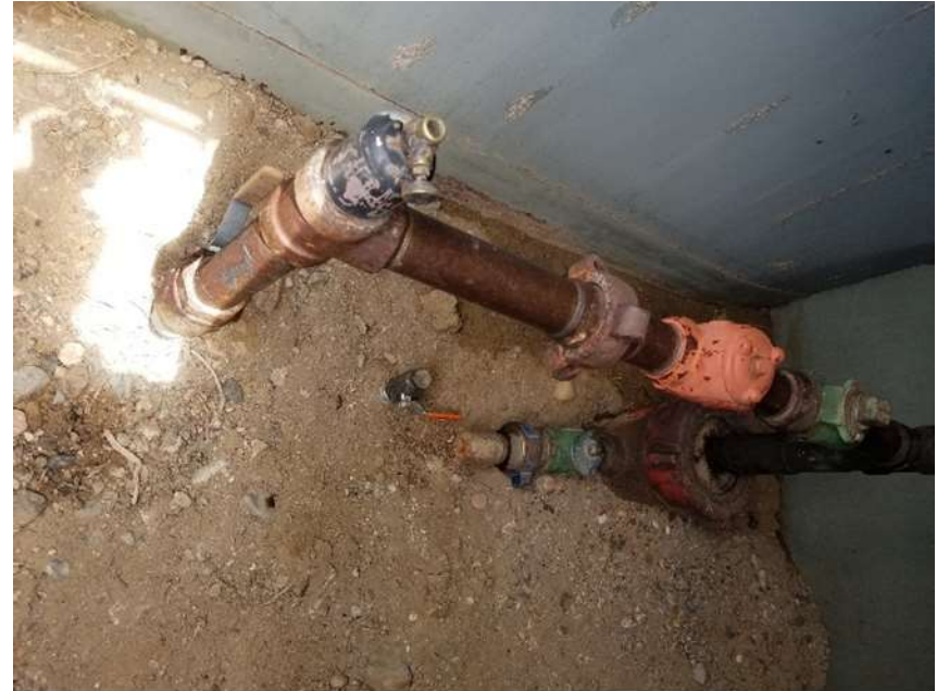
Photo 2. Close up of wellhead inside housing.
