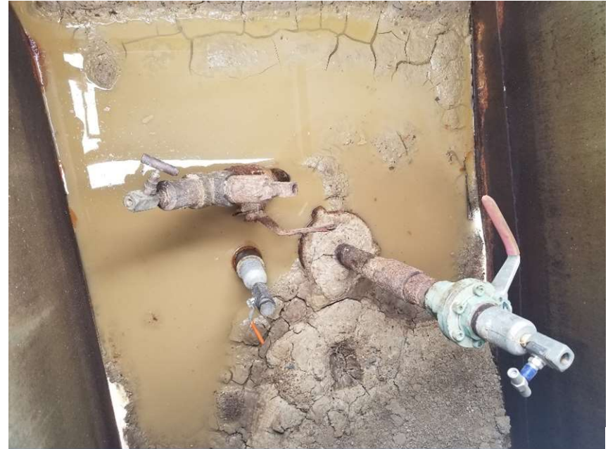
Photo 2. Photo of wellhead inside housing cover.
