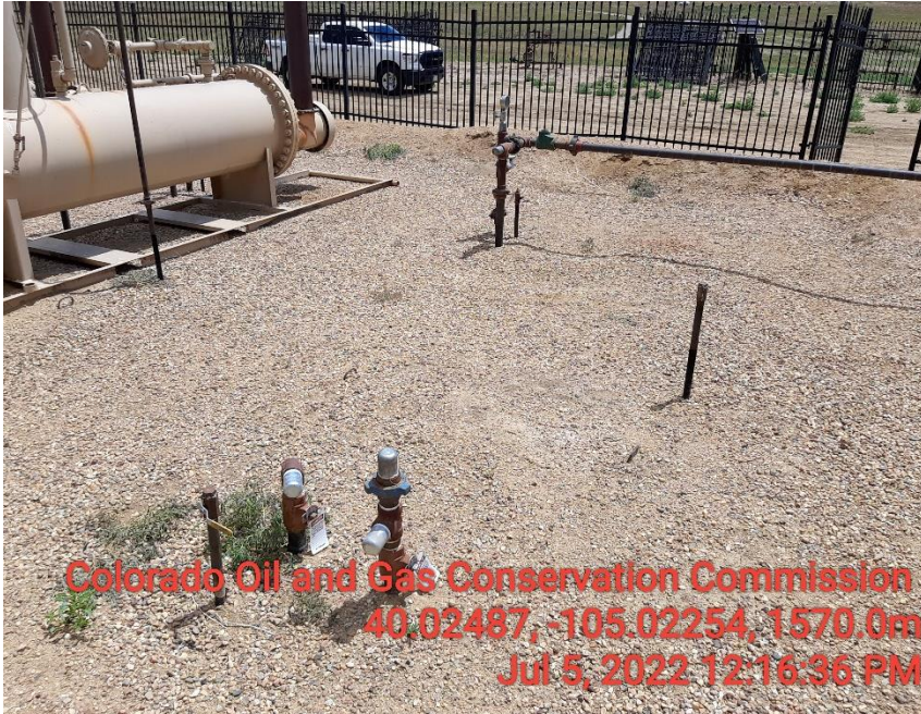
Photo 7 flow lines not LOTO. Tag have no writing
