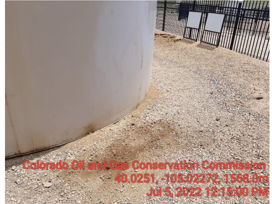
Photo 6 Stained soil around crude oil tank.
