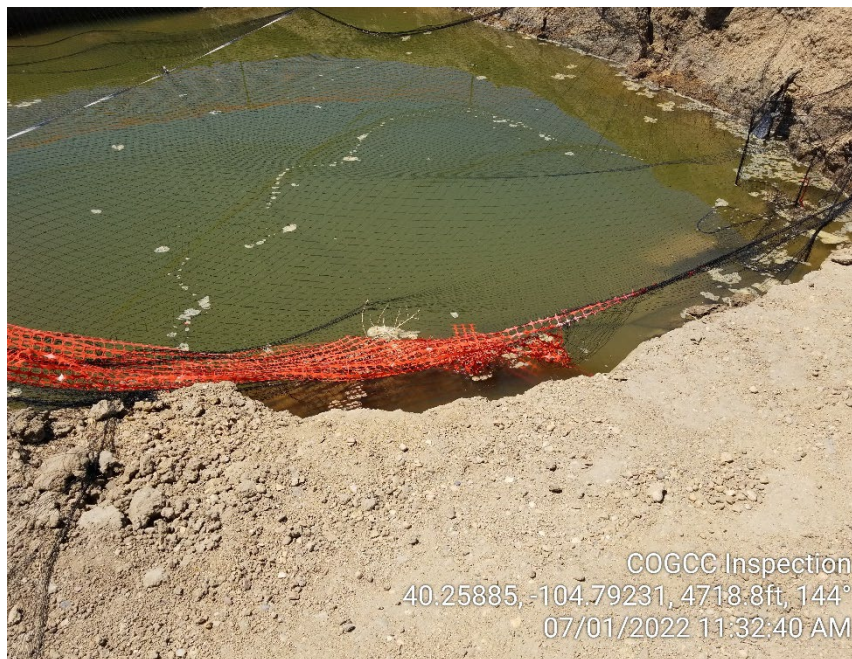
Photo 3 – Downed fencing in open excavation.
