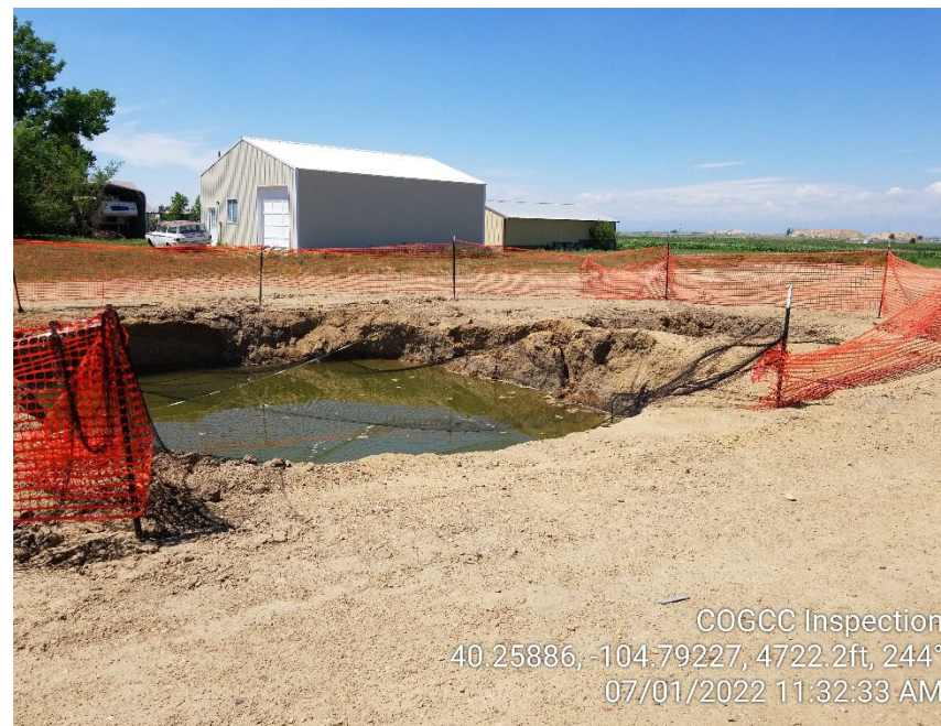
Photo 2 – Location photo. Fencing is down. Groundwater observed in open excavation. Groundwater is covered with bird netting.
